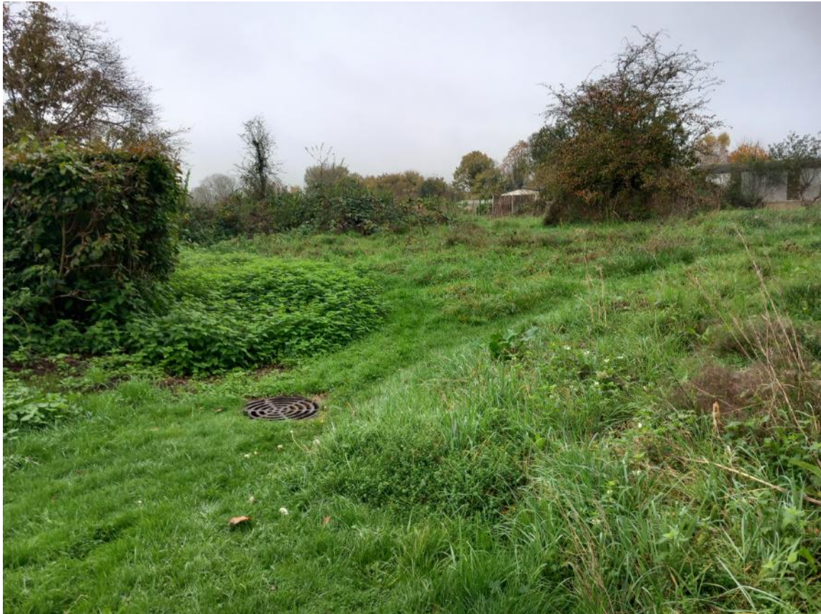
Plate 7: Drain cover located near Moor Lane, c.35m southeast of the proposed route. Photograph taken facing west.
