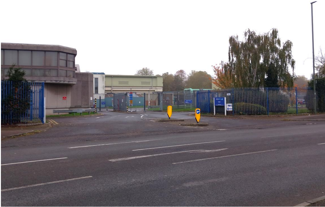
Plate 1: Affinity Water Limited compound on the northern side of The Causeway. Photograph taken facing northeast.
