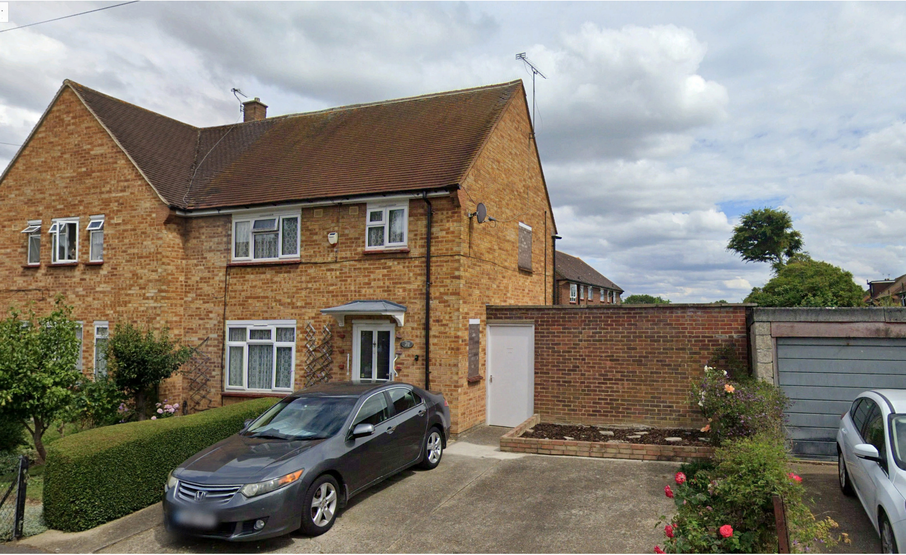
Existing Front View
