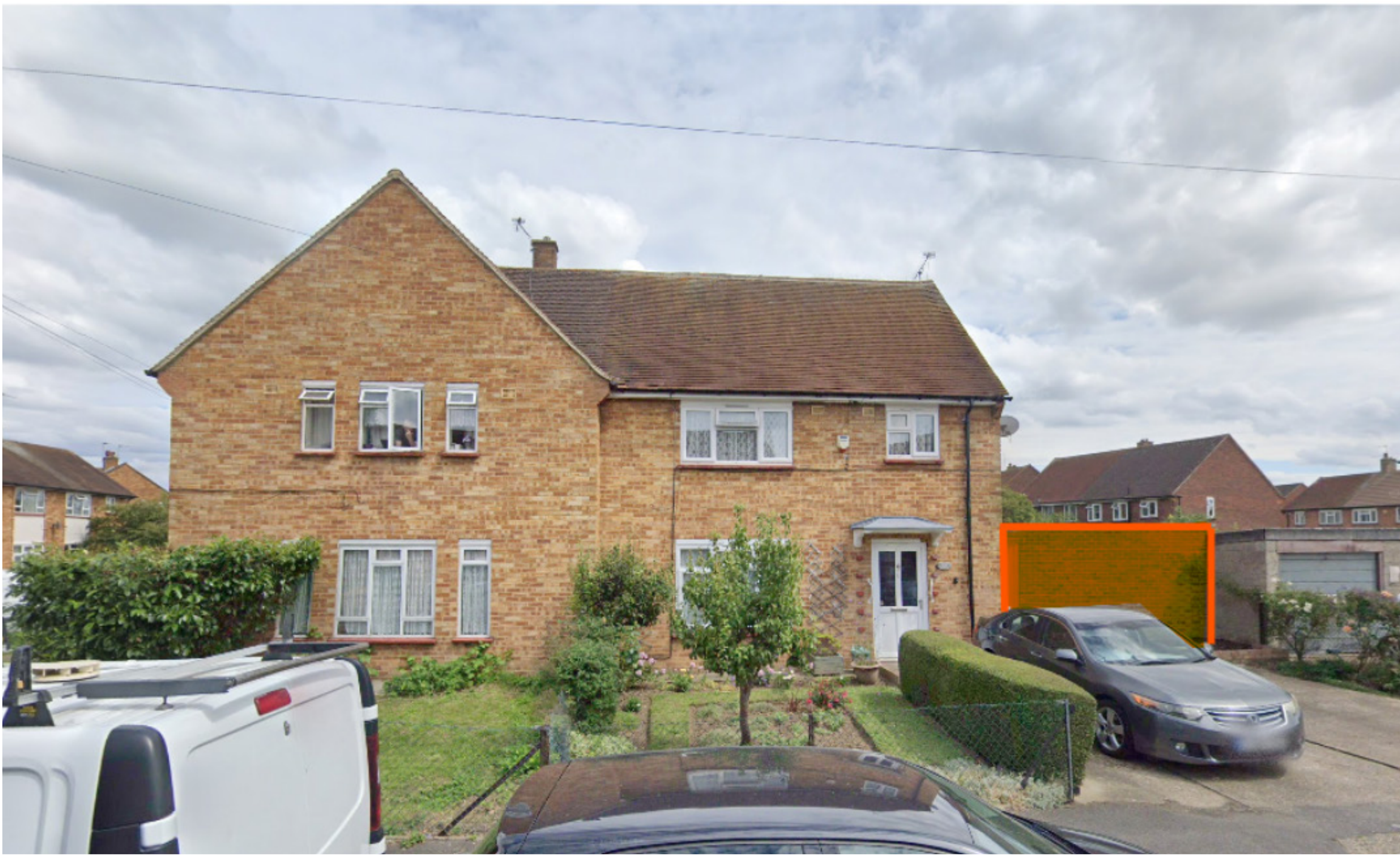
Existing Front View
