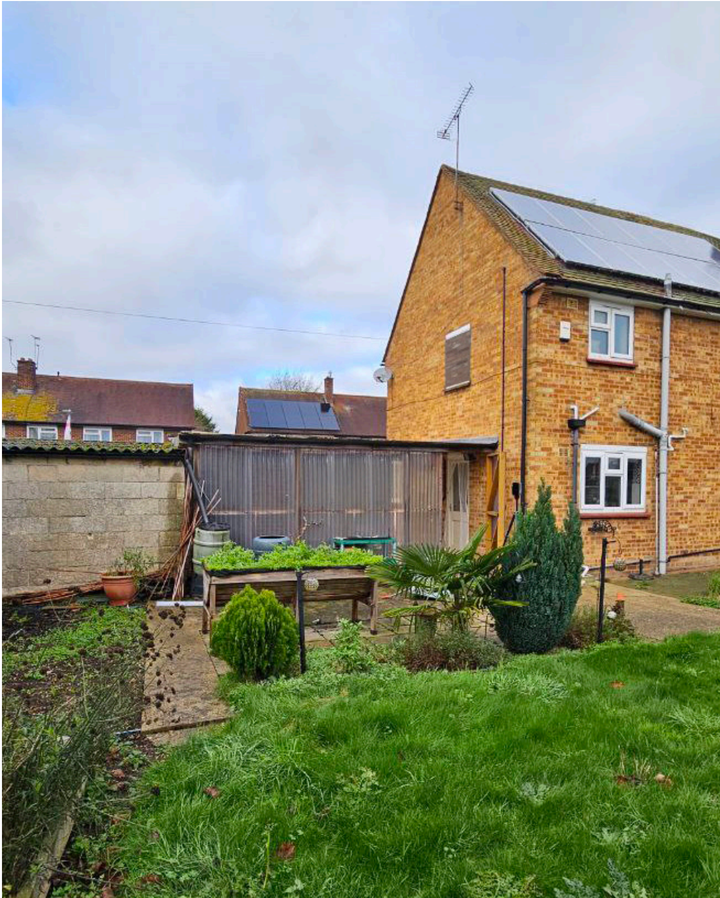
Existing Rear View
