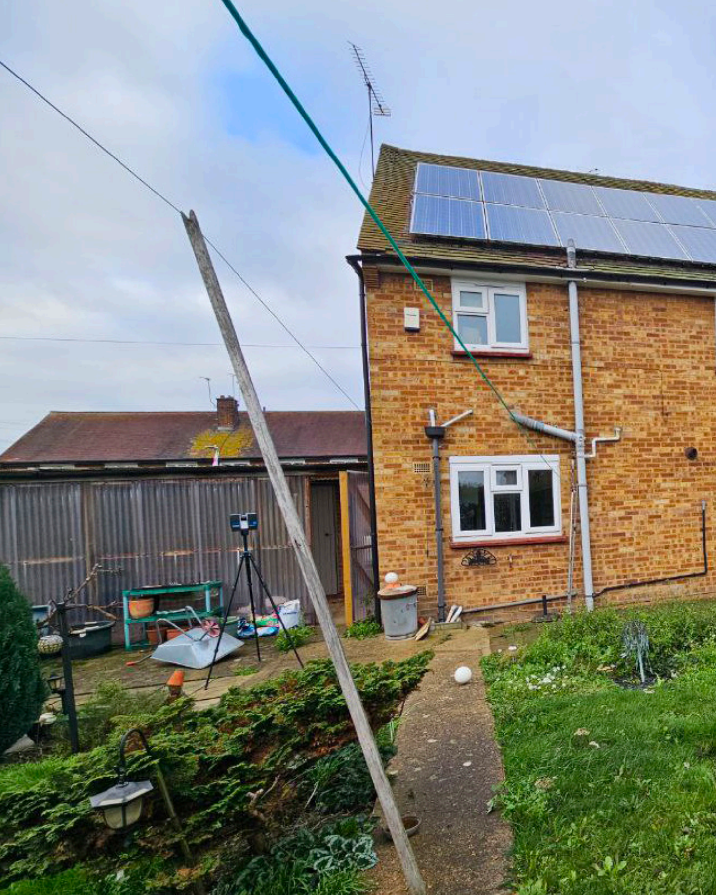
Existing Rear View
