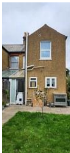
The rear elevation of the host dwelling at No. 1 South Walk, where the approved 3.6m rear extension will be constructed
