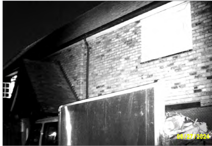
Photograph of northern elevation of Building 4 at end of survey 3
