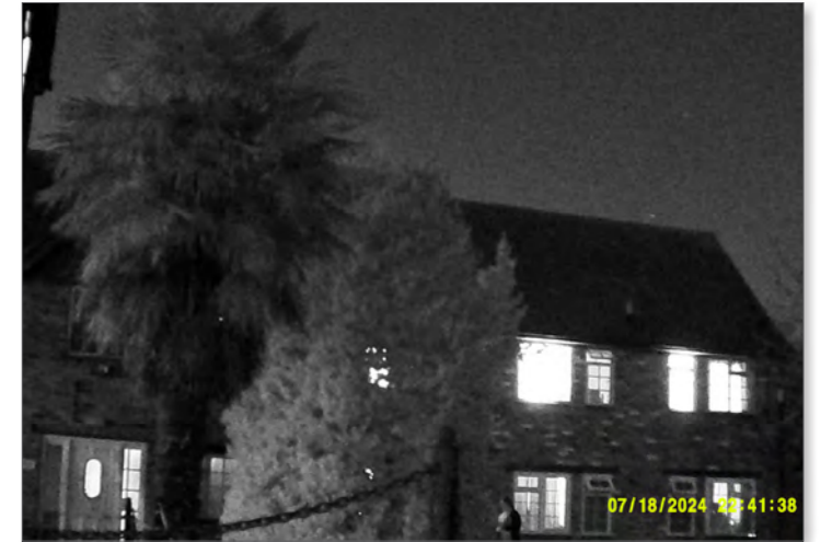
Photograph of eastern section of the southern elevation of Building 4 at end of survey 4
