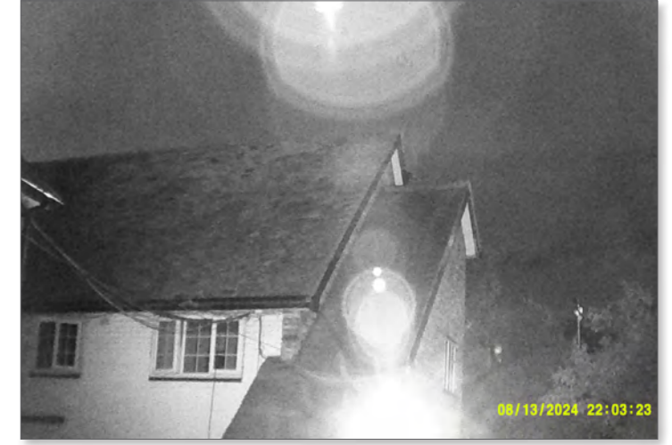
Photograph of the northern and eastern elevations of Building 3 at the end of survey 5.
