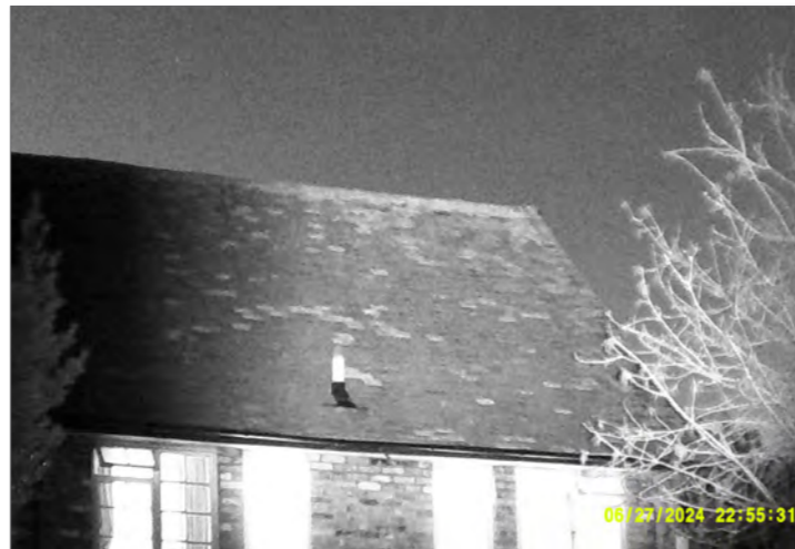
Photograph of southern elevation of Building 4 at end of survey 3
