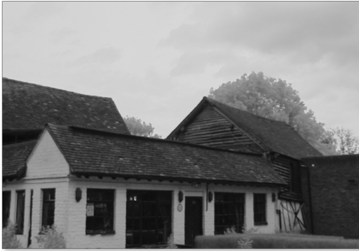
Photograph of northern and western elevations of Building 1 at start of survey 2
