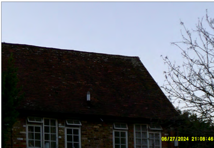
Photograph of southern elevation of Building 4 at start of survey 3
