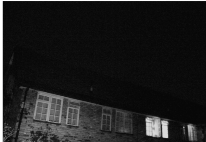
Photograph of western section of the southern elevation of Building 4 at the end of survey 4
