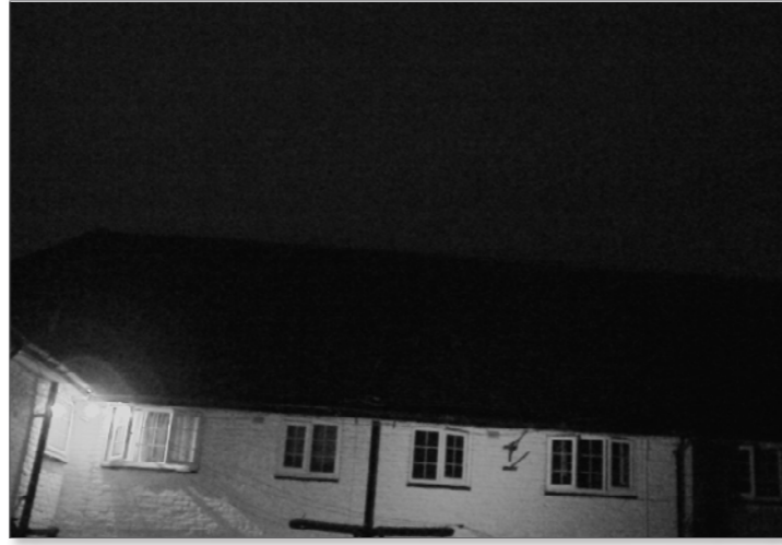
Photograph of the eastern elevation of the northern section of Building 3 at the end of survey 5.
