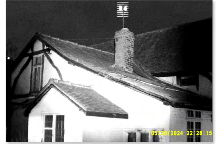
Photograph of southern and eastern elevations of Building 2 at end of survey 2
