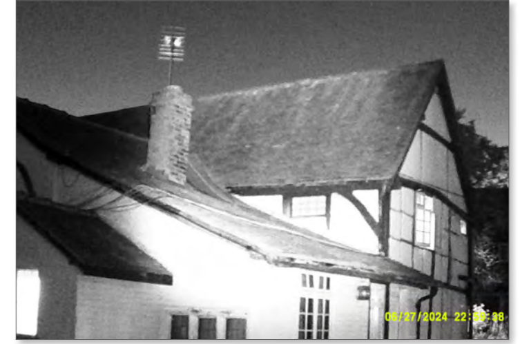
Photograph of southern and eastern elevations of Building 2 at end of survey 3
