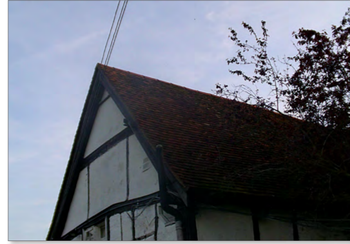
Photograph of northern and eastern elevations of Building 2 at start of survey 1
