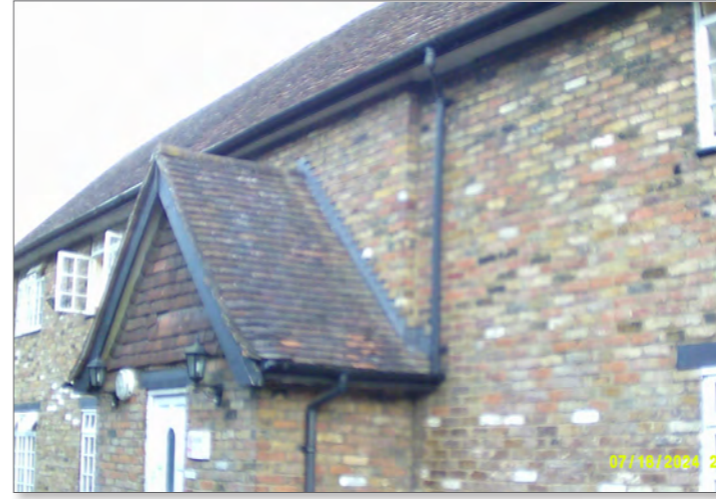
Photograph of northern elevation of Building 4 at start of survey 4
