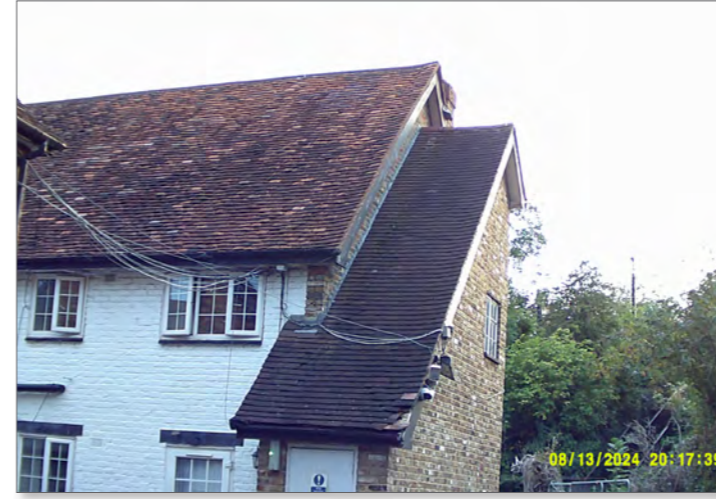
Photograph of the northern and eastern elevations of Building 3 at the start of survey 5.
