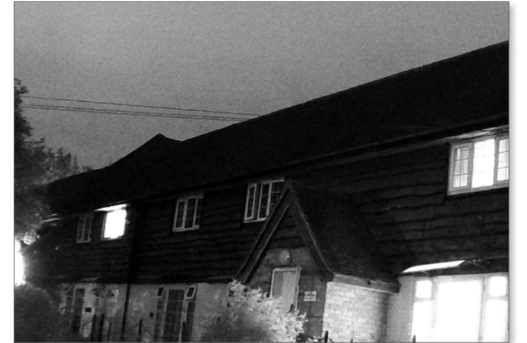
Photograph of eastern section of the southern elevation of Building 3 at end of survey 2
