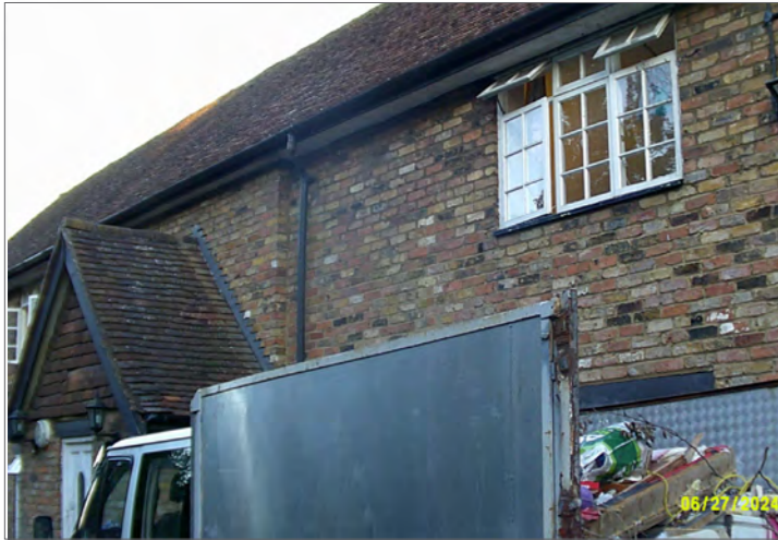
Photograph of northern elevation of Building 4 at start of survey 3
