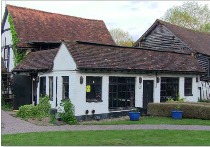
Photograph of northern and western elevations of Building 1 at start of survey 1
