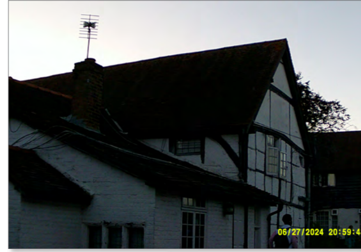
Photograph of southern and eastern elevations of Building 2 at start of survey 3
