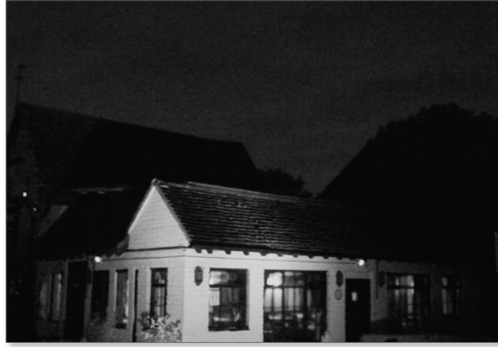
Photograph of northern and western elevations of Building 1 at end of survey 2
