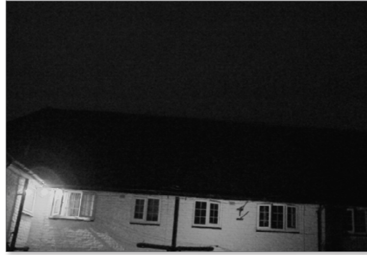
Photograph of the eastern elevation of the northern section of Building 3 at the end of survey 5.
