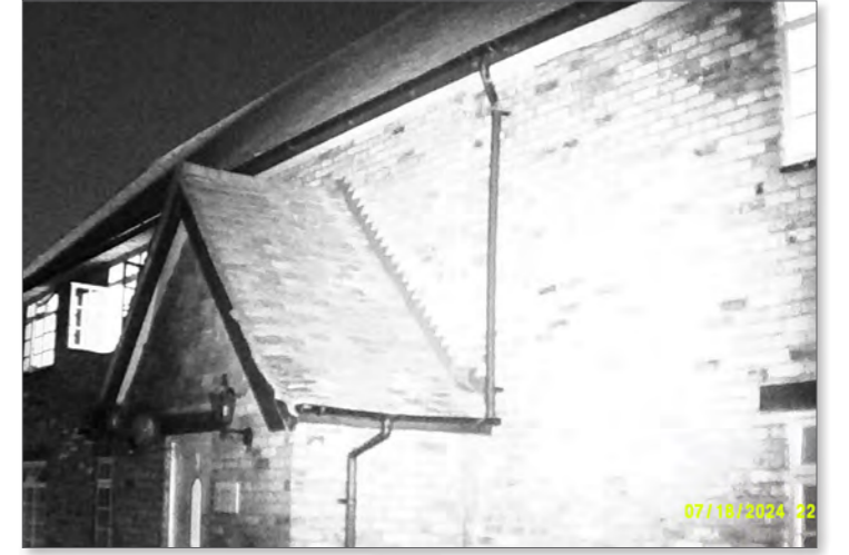
Photograph of northern elevation of Building 4 at end of survey 4
