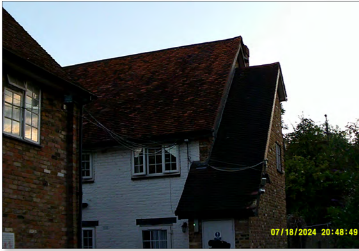
Photograph of northern and eastern elevations of Building 3 at start of survey 4
