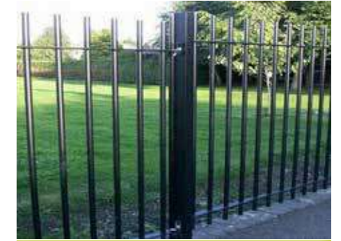
1.8m High Metal Railing
