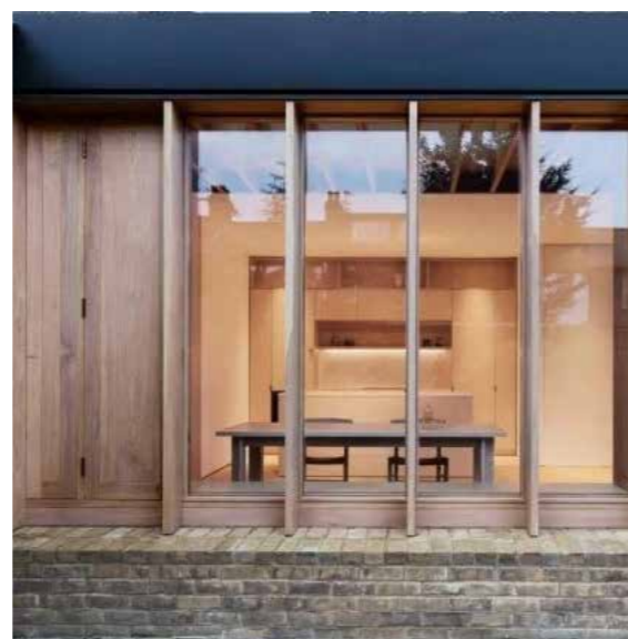
Figure 4.17: Ribbed Timber Frame / Glass
