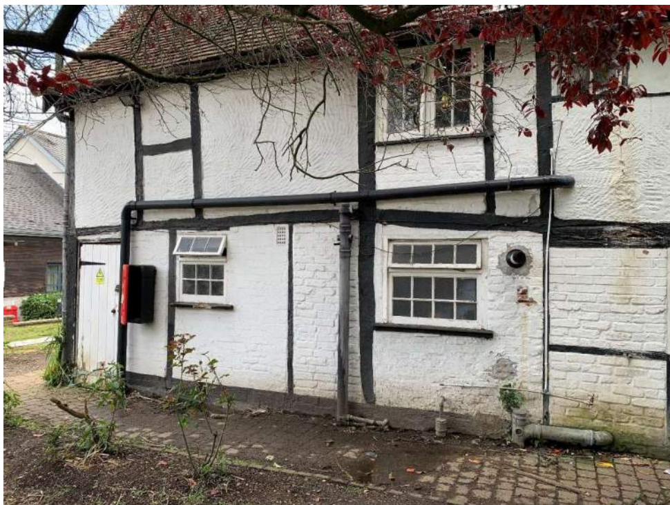
Photograph 6 – North elevation eastern end
