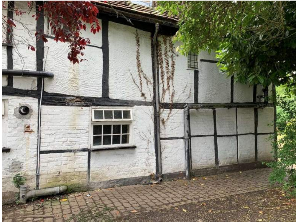
Photograph 7 – North elevation western end
