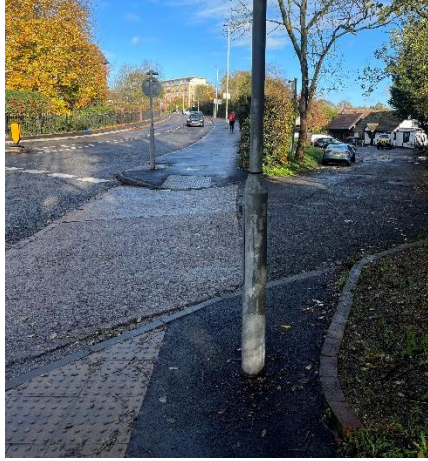
Photograph 1: Existing Conditions West End Road northbound
