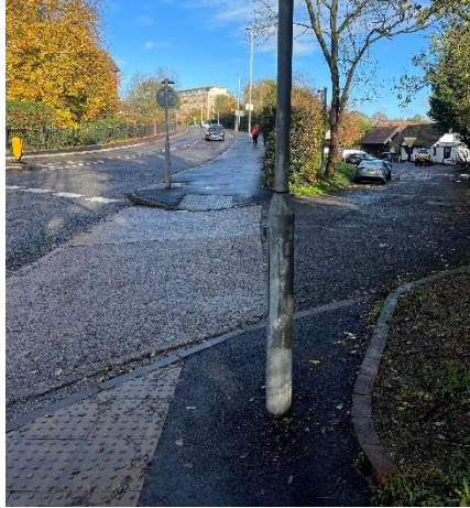
Photograph 1: Existing Conditions West End Road northbound
