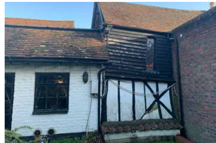
Figure 5.6 Twentieth-century additions to the barn buildings shown buttressing a historic section of the Leaning Barn which is in a state of disrepair
