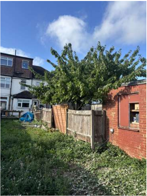
6. View showing adjoining building no.33
