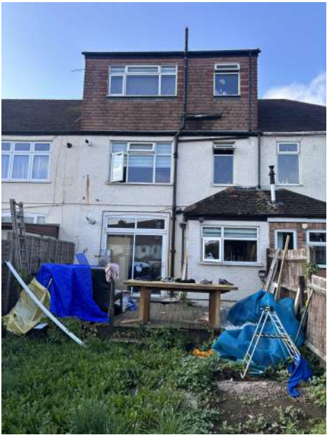
4. View of the rear of the house
