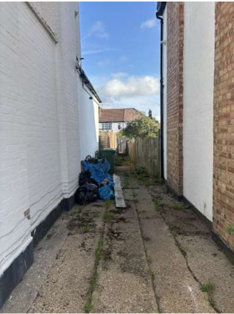
7. Alley way to the rear of garden
