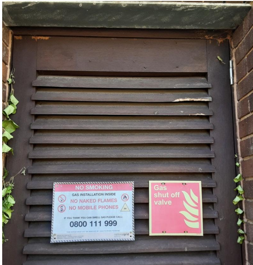
Photograph 13: PRF4 – Space between wooden beams provides access for bats into interior of building
