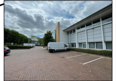
PH05: View of southern office building.
