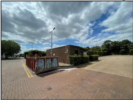
PH03: View of skip and southern sub-station.
