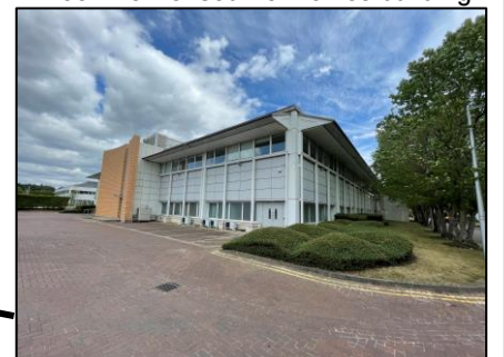
PH06: View of southern office building.
