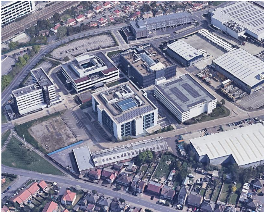
Figure 1: Oblique aerial photograph of the site looking north-west (Source: Google)
