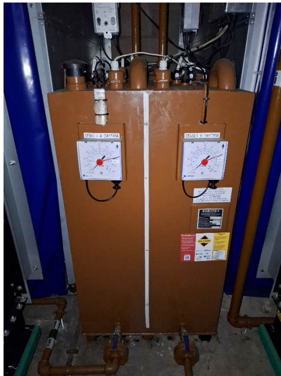
Photo 4. View of diesel day tanks in substation/ generator building
