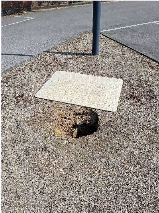
Photo 25. View of area of ground instability on 'island' in the surface car park in the north of the site
