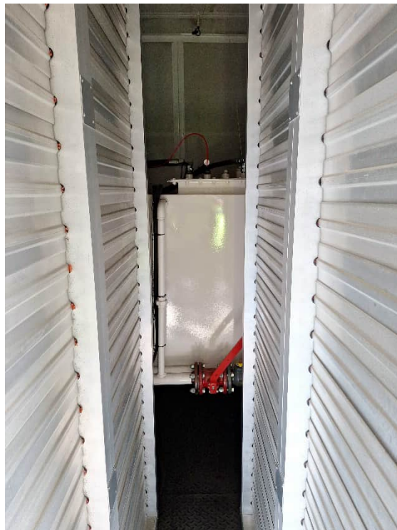
Photo 10. View of back-up generator diesel day tank for HPH5 building
