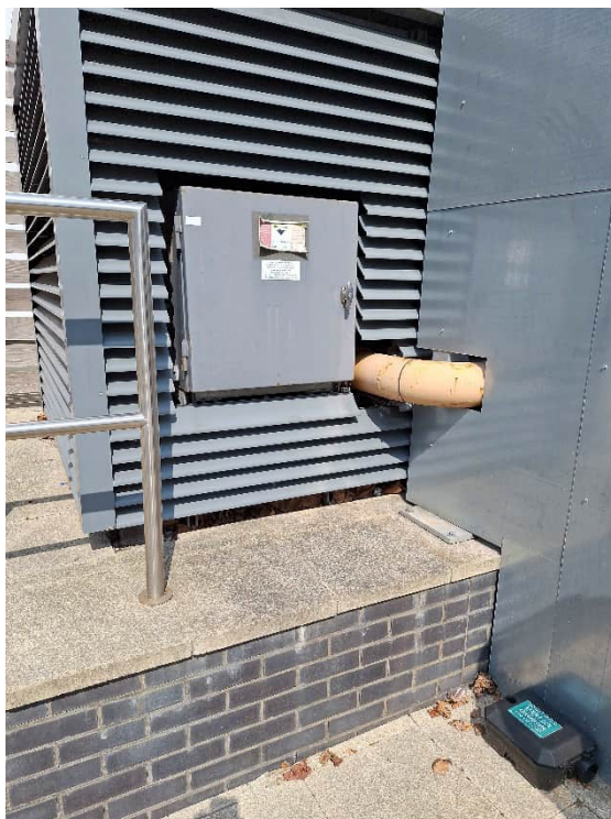
Photo 16. View of main diesel tank fill point on external wall of HPH5 building
