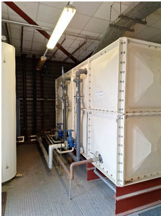
Photo 18. View of rooftop cold water storage tank for HPH2
