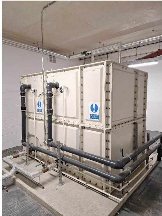
Photo 7. View of cold water storage tank in basement of HPH5 building
