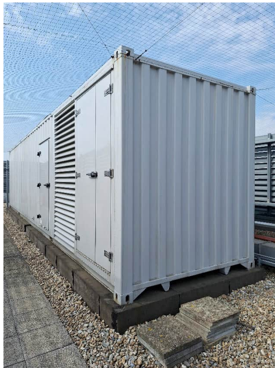
Photo 8. View of rooftop backup generator and diesel tank container for HPH5 building
