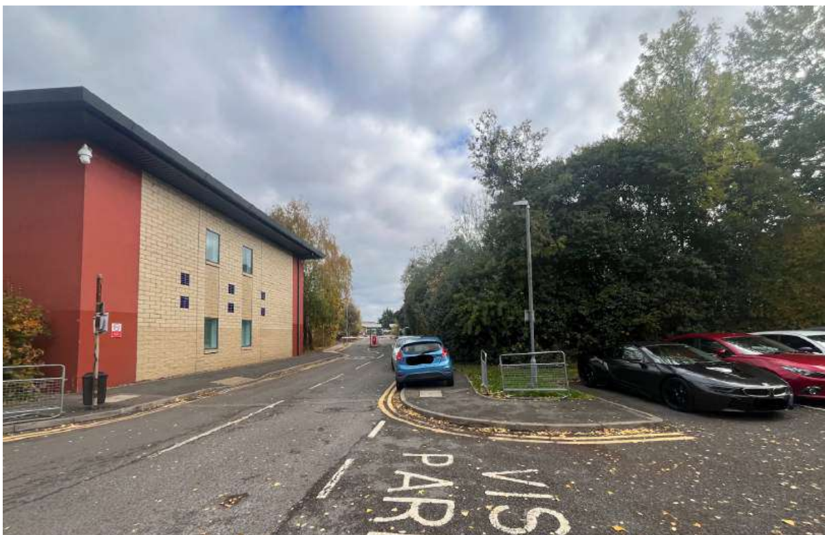
5 - South of the Site facing East.
