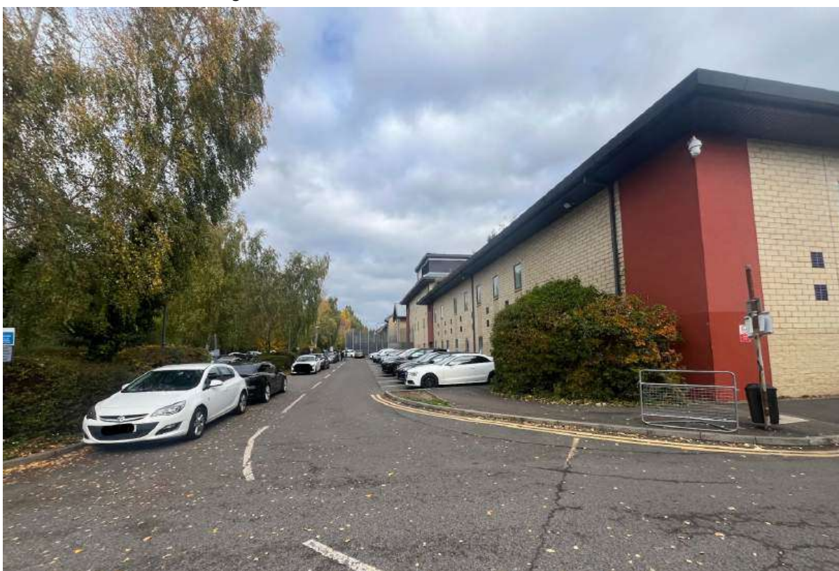
6 -South of the Site facing North, depicting H11 and H9.
