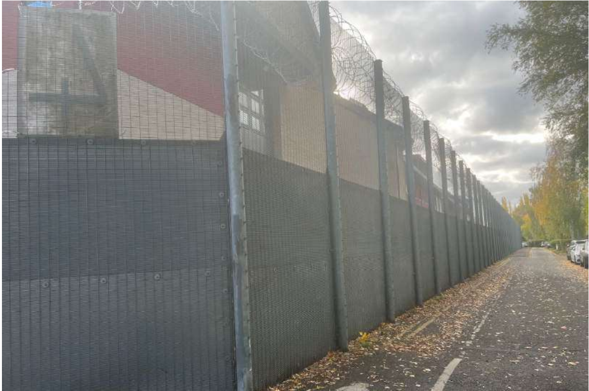
29 - Northern section of the site facing South-West.
