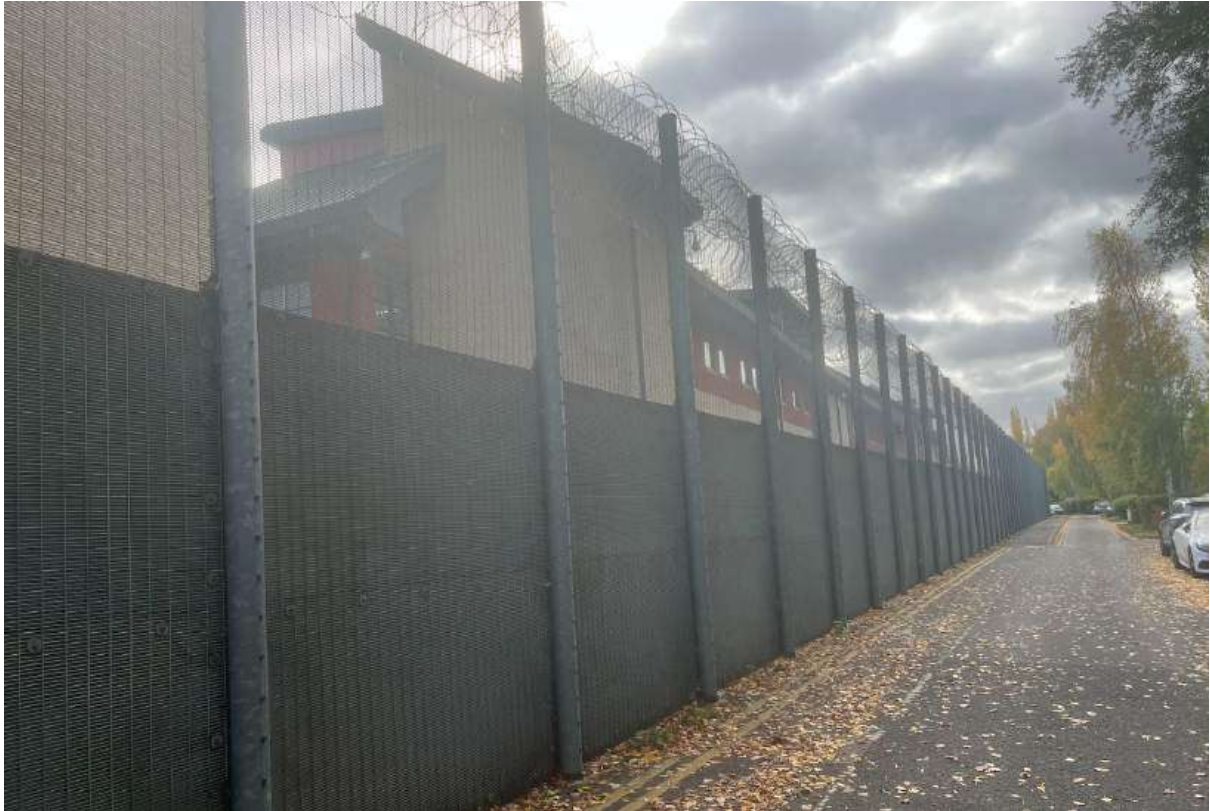
27 - Central section of the site facing South-East.
