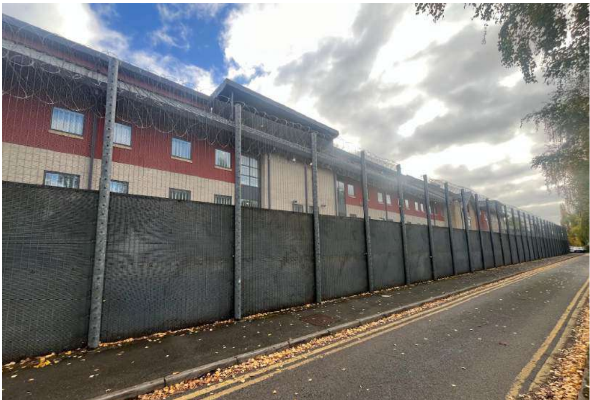
23 - Central section of the site facing South-East.
