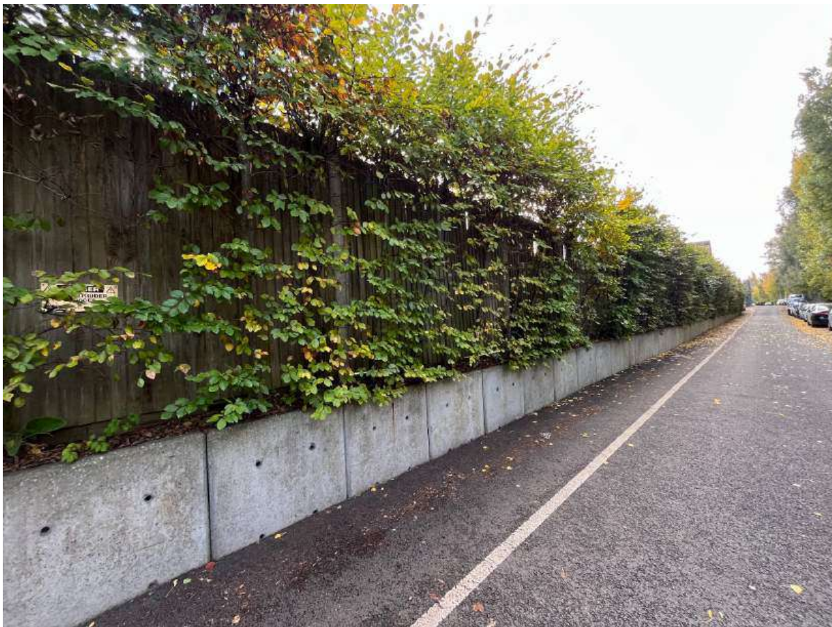
37 - Northern section of the site facing South-East.
