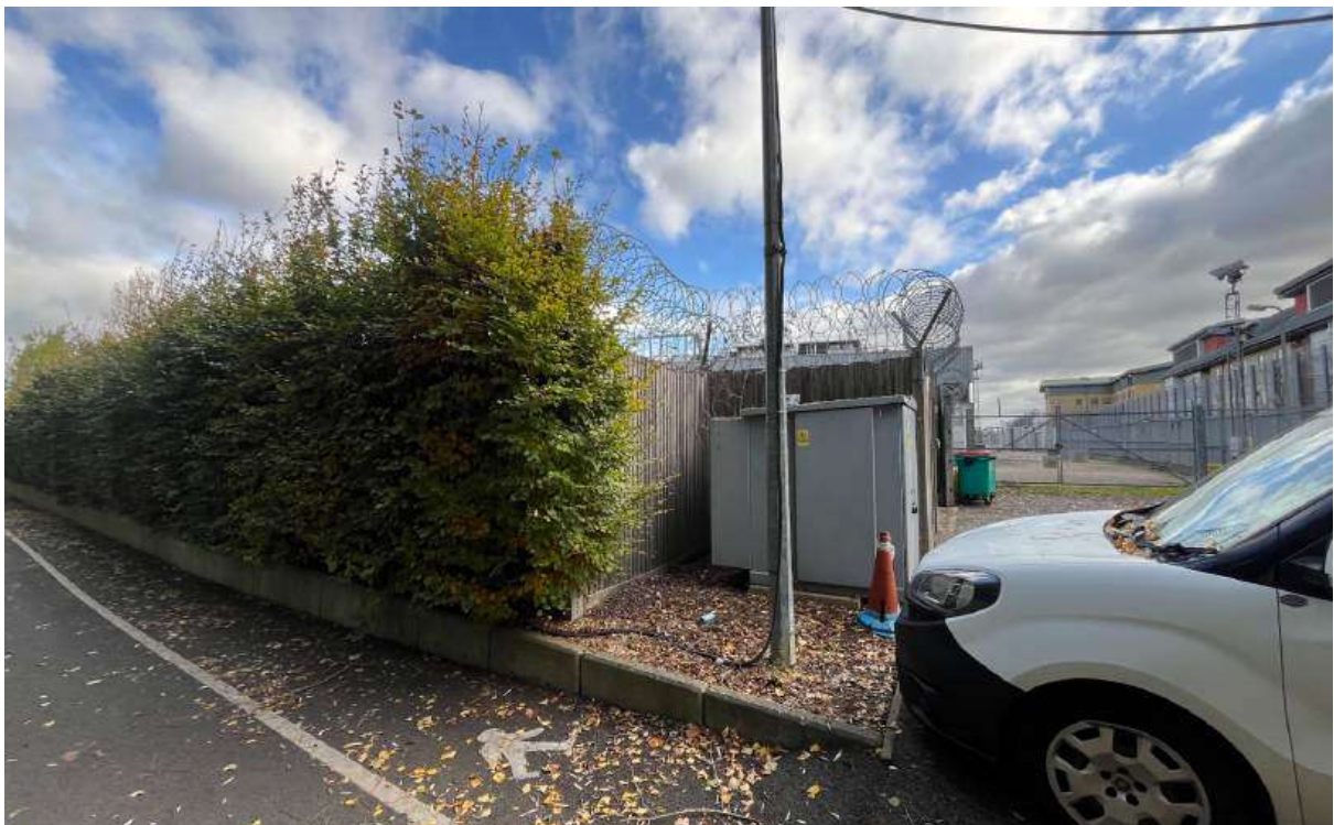
32 - Northern section of the site facing East.
