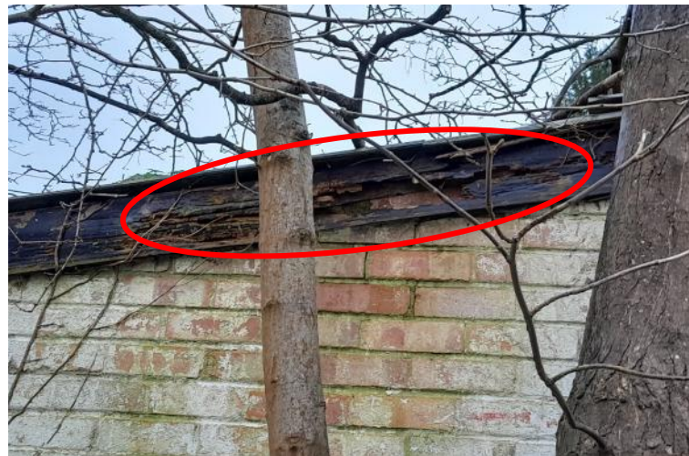
Figure 22 - View of gap in barge board on B2.
