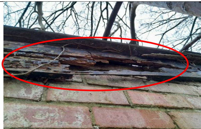
Figure 23 - View of gap in barge board on B2.
