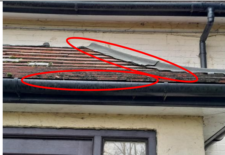
Figure 10 - View of gaps beneath tiles and flashing on the porch.
