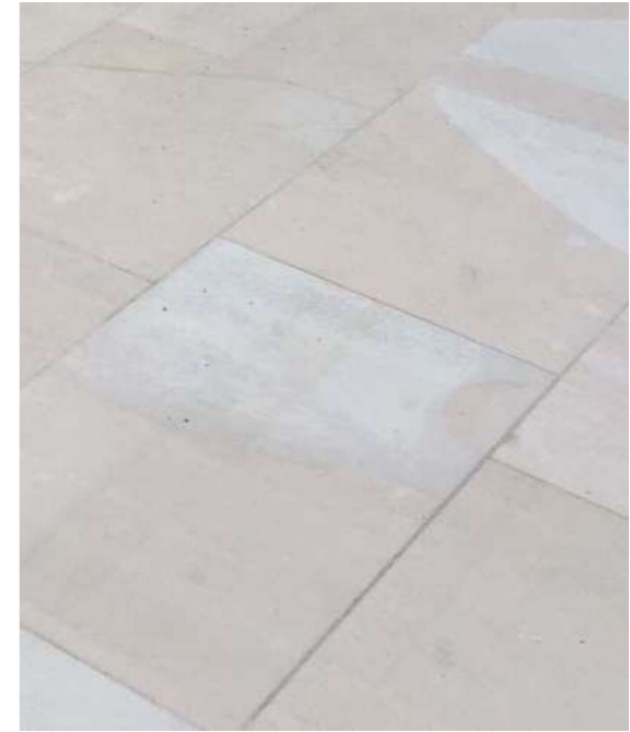
Large format sawn Limestone paving will be used to indicate the entrances to the individual homes and be used for generous terraces to the rear of each property
