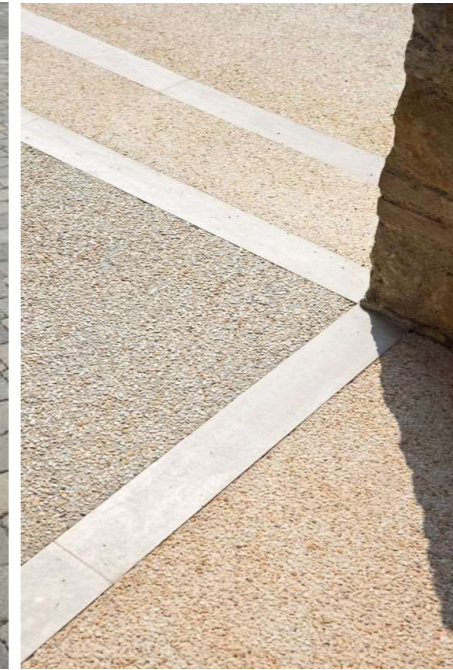
SUDS compliant resin bound gravel will be used in the shared pedestrian zones
