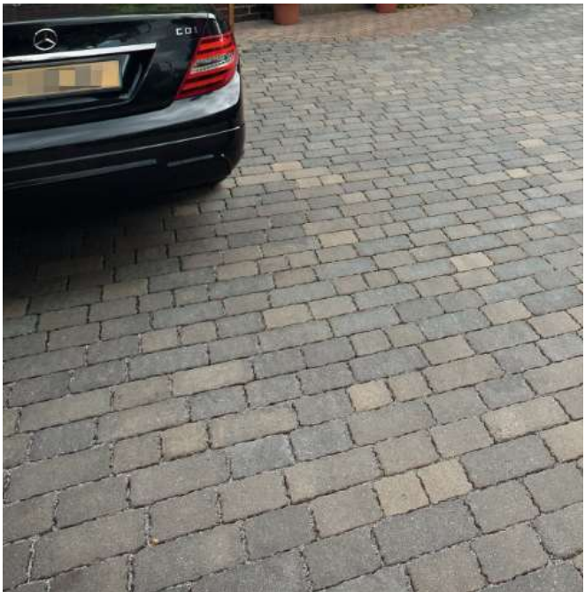
SUDS compliant permeable block paving to the entrance and parking areas will help to manage heavy rainfall in a sustainable way, with surface water passing through into the ground below.
