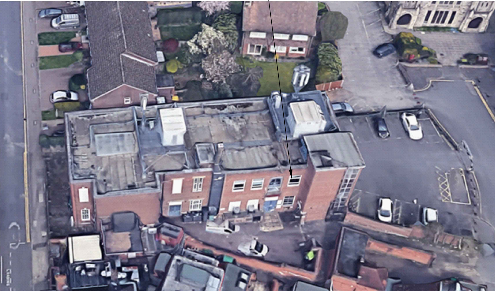
AERIAL VIEW OF SOUTH ELEVATION
