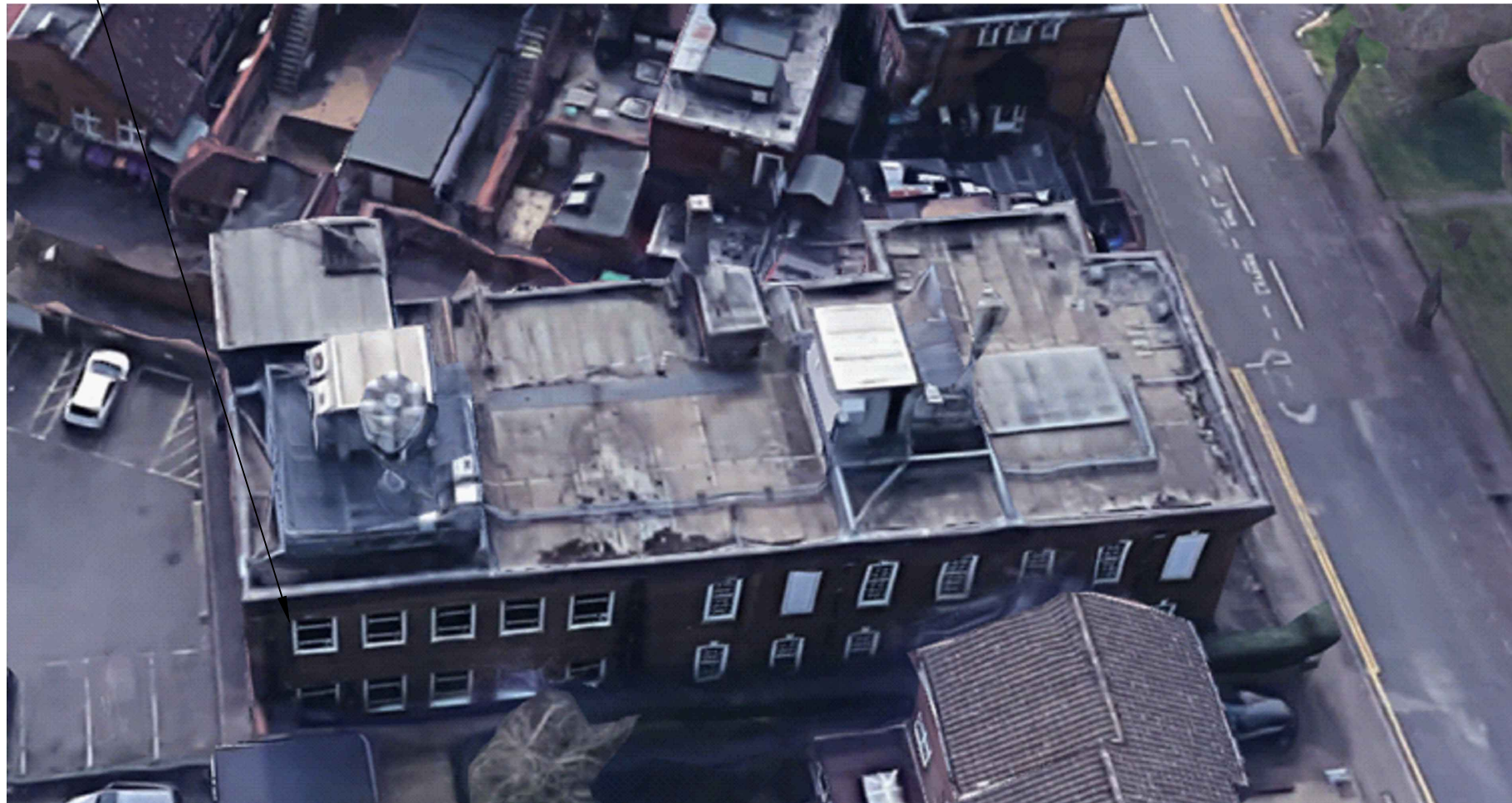
AERIAL VIEW OF NORTH ELEVATION
