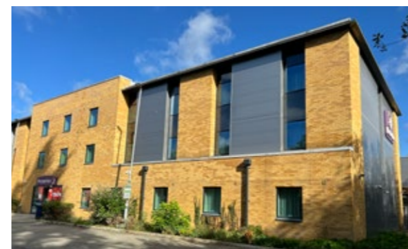
View from Car Park
