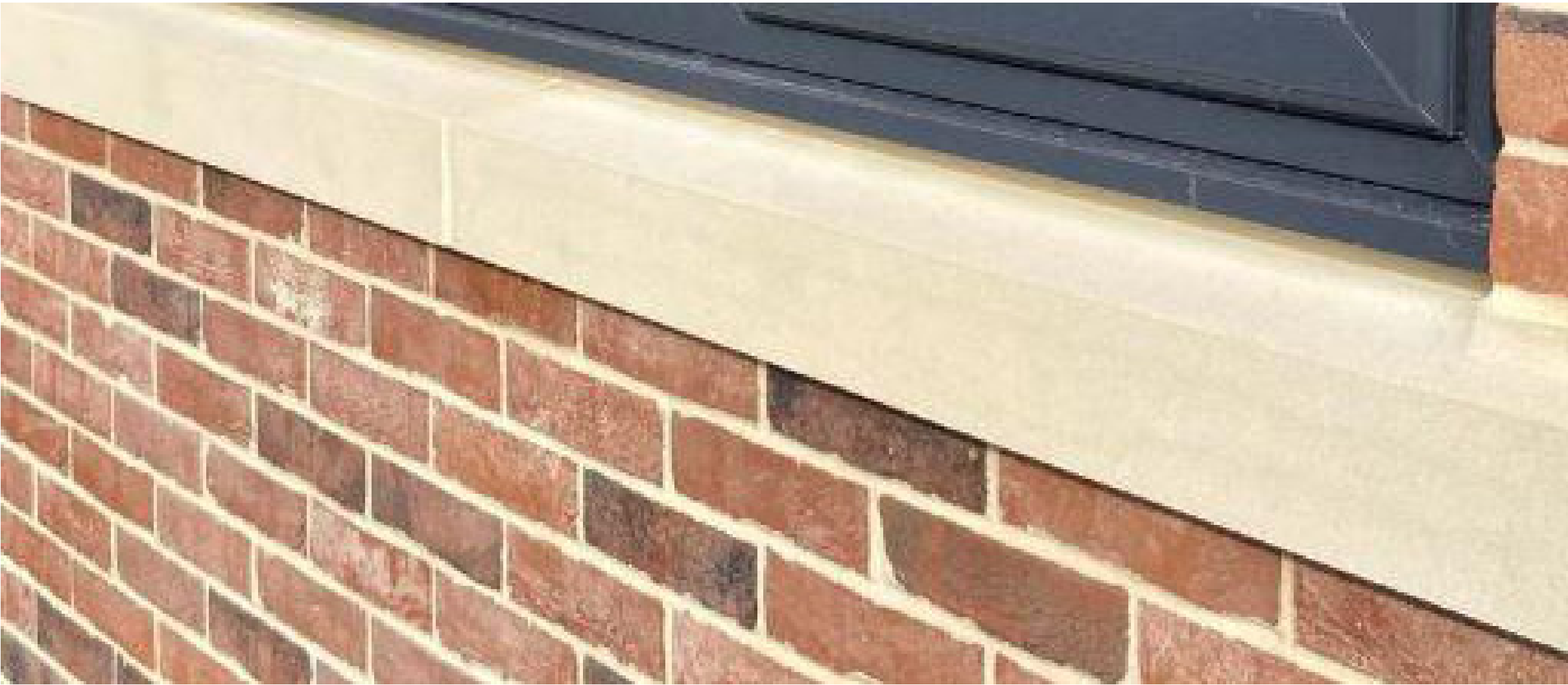
precast concrete window sills
