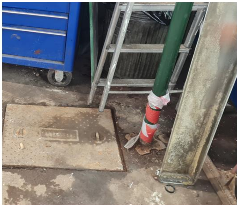
Photo No.5: Manhole covering noted in concrete-flooring of the garage unit, some staining noted around the feature
