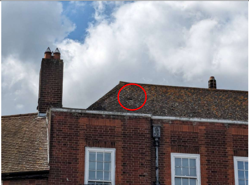
Photo 2. – View of the northeast roof elevation and missing tile.
