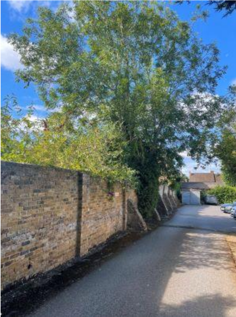
Ash tree viewed from access road to car park, showing retaining wall and buttresses.
