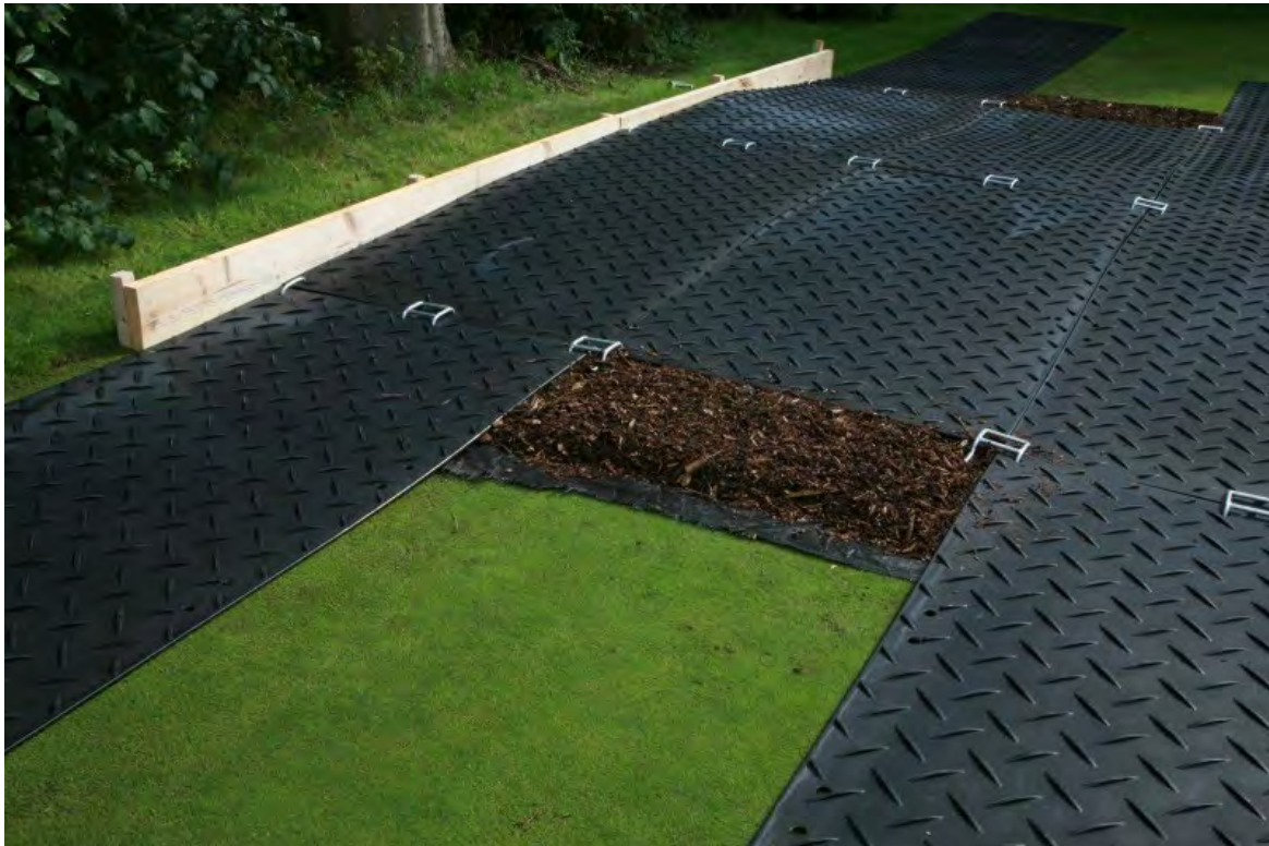
Figure 3. Example of propriety inter-linked ground protection boards placed on top of a compression-resistant layer (e.g. 150 mm depth of woodchip), laid onto a geotextile membrane, suitable for pedestrian-operated plant up to a gross weight of
