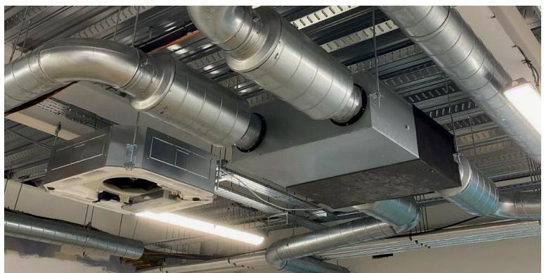
The MVHR units shall be in the ceiling void. Each unit shall draw fresh air and discharge extract through the façade. The intake and exhaust louvers shall be separated to prevent cross contamination with a filter inside the unit near the heat exchanger to remove pollen and particulate matter.
