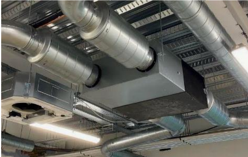
Typical Exposed MVHR configuration
