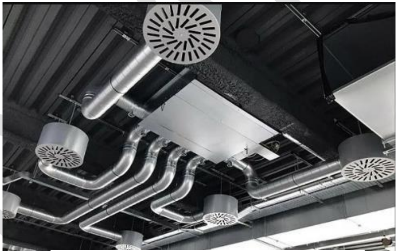
Typical VRF Fan Coil to Amenity Spaces
