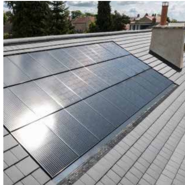
Roof mounted PV panels
