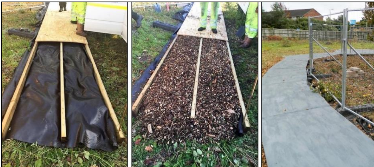
Image 8: Showing an example of a ply boarding above woodchip system of temporary ground protection.
