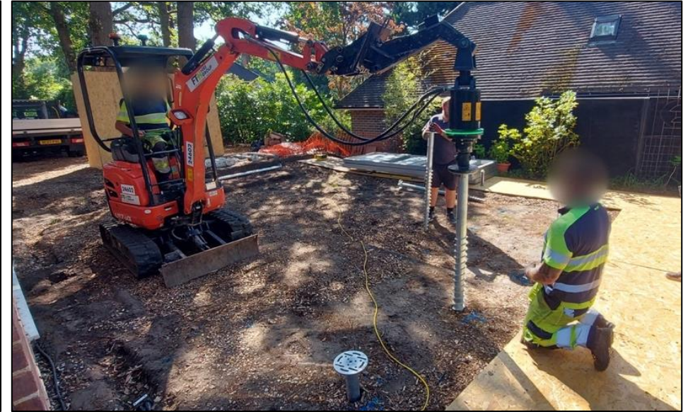
Image 15: Showing ground screw pile installation.
