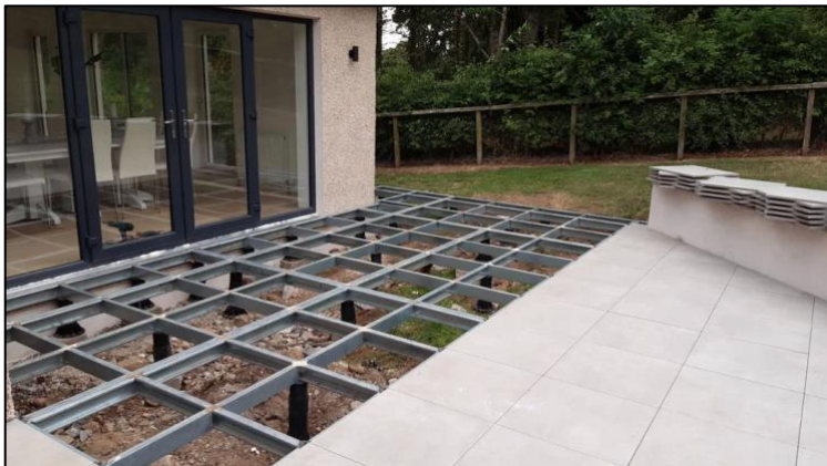
Image 13: Example of a modular paving subframe (Tectonic®).
