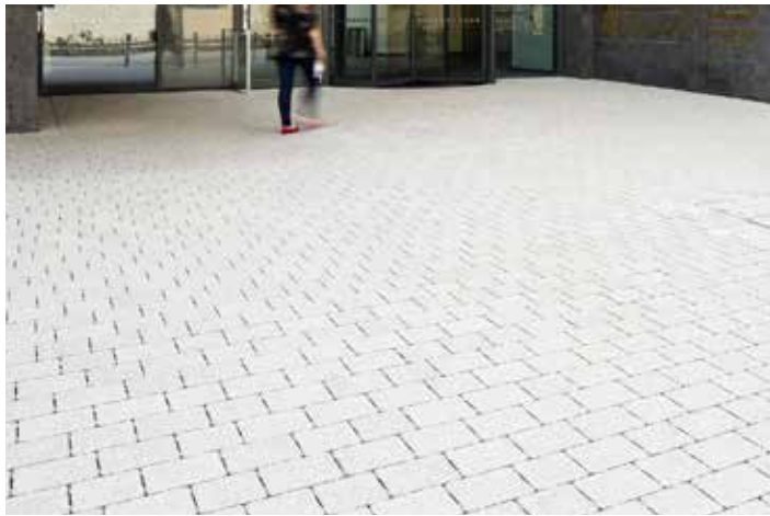
Example of Permeable Paving - Laid in stretcher bond Silver Grey colour
