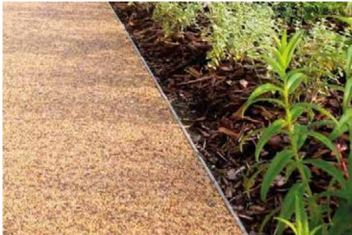
Metal edging to define planting areas between hard and soft surfaces
