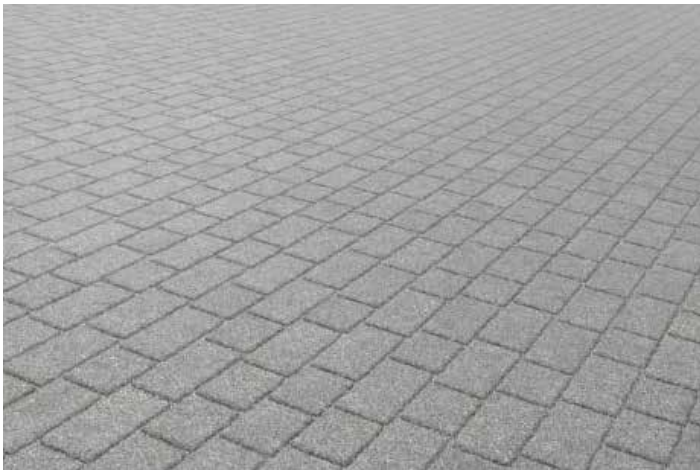
Example of Permeable Paving - Laid in stretcher bond Mid grey colour
