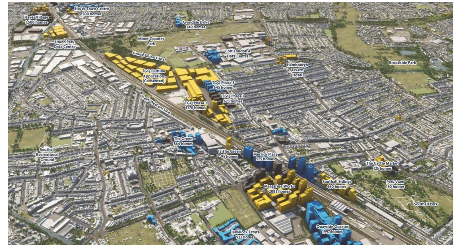
Image 2.2.7.3. Green Quarter aerial view in context, image produced in VuCity, by JTP Arch.
