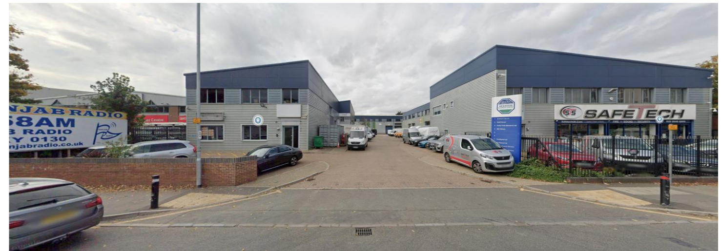
Image 2.2.1.4. Google Maps view of Safe Tech building along Springfield Rd.
