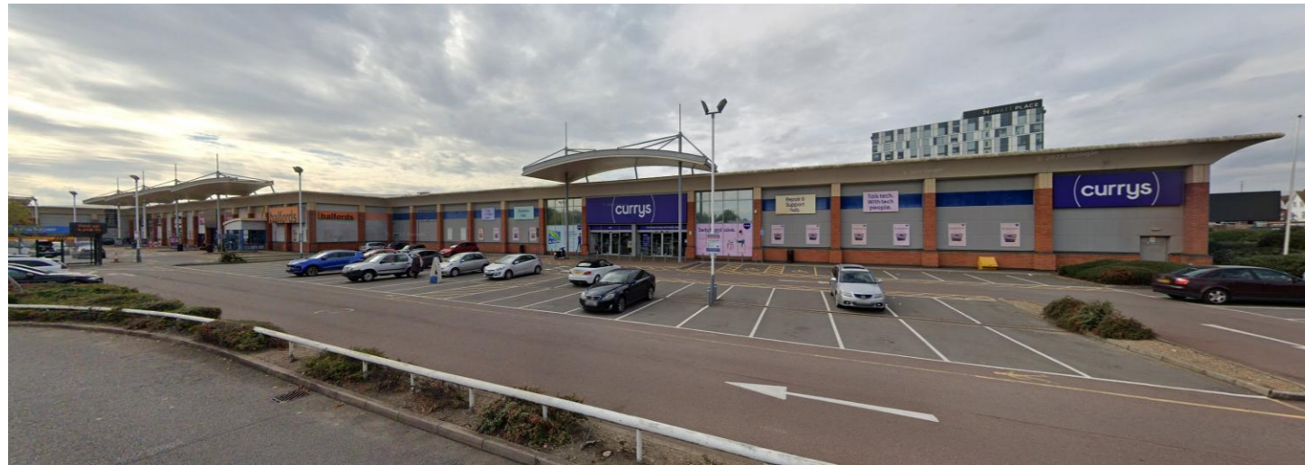
Image 2.2.2.1. Google Maps view of Hayes Bridge Retail Park
