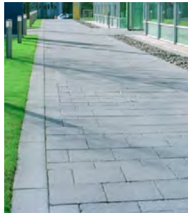
Block paving footways
