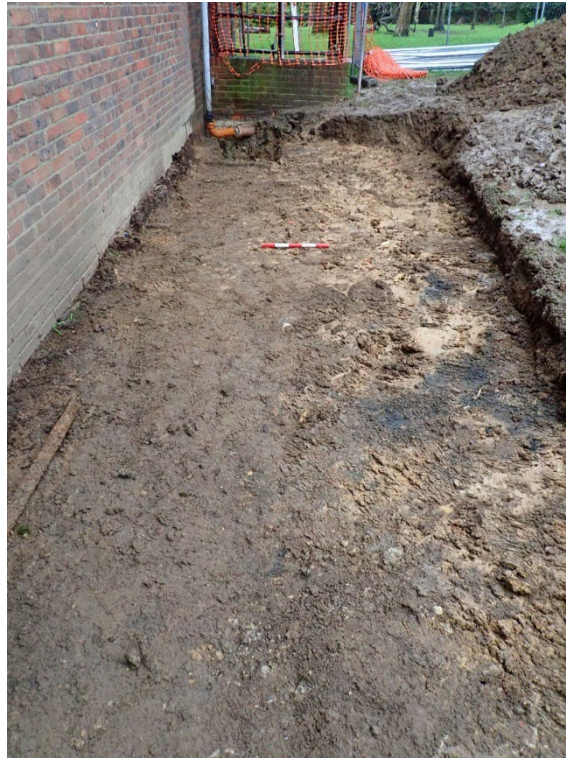
Plate 6: Foundation trench looking north showing transition to reworked clay [1] below modern made ground.
