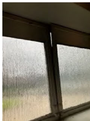
Figure 57. Metal frame window unable to close
