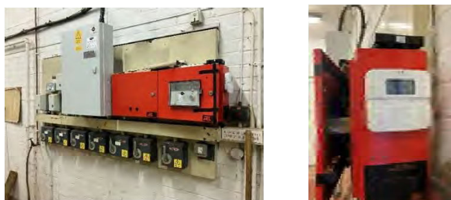
Figure 64. Obsolete BMS and simple time schedule controllers
