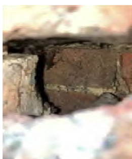
Figure 70. Winston Churchill Theatre, brickwork damage during stage deliveries
