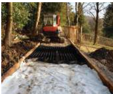
Fallbarrow Park, Windermere: CellWeb TRP® Installation
