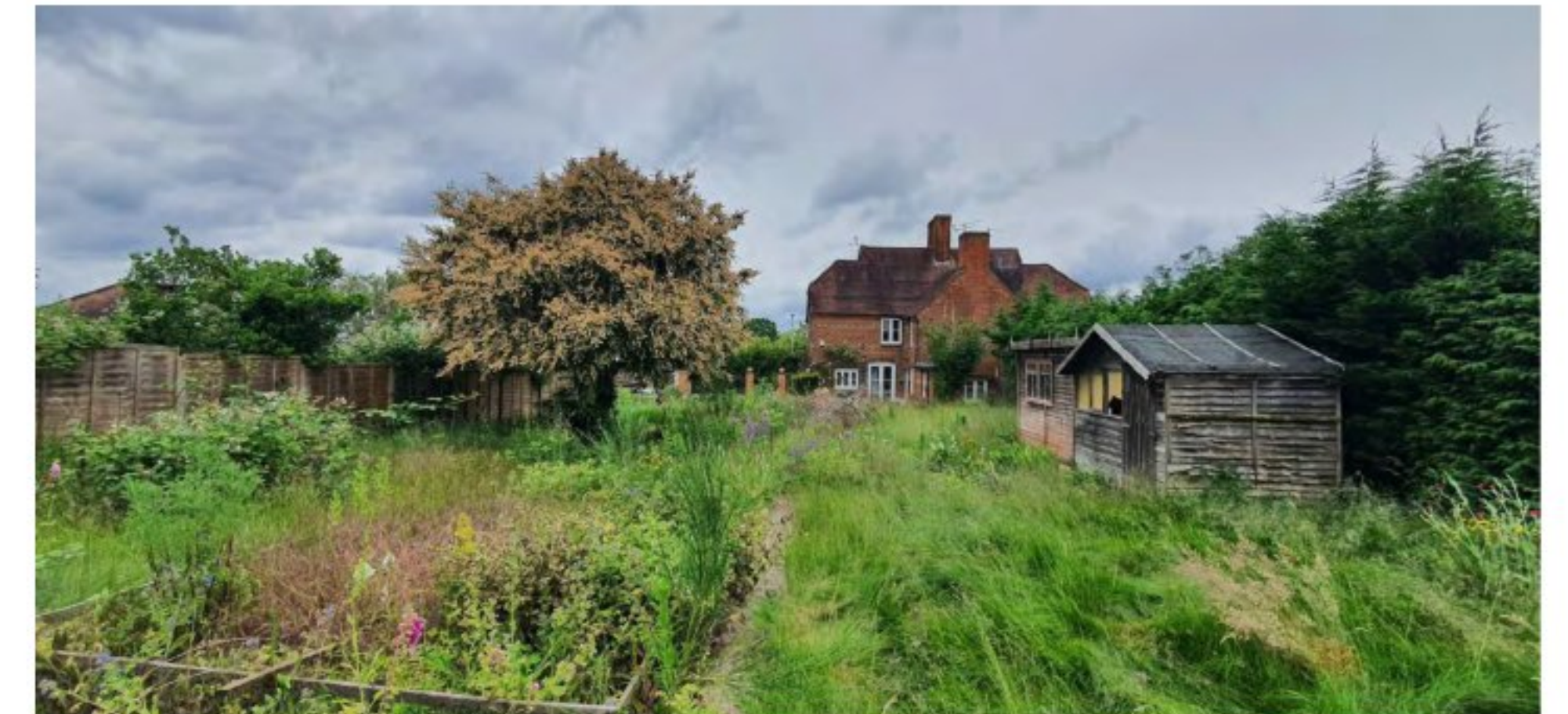
View towards front of site
