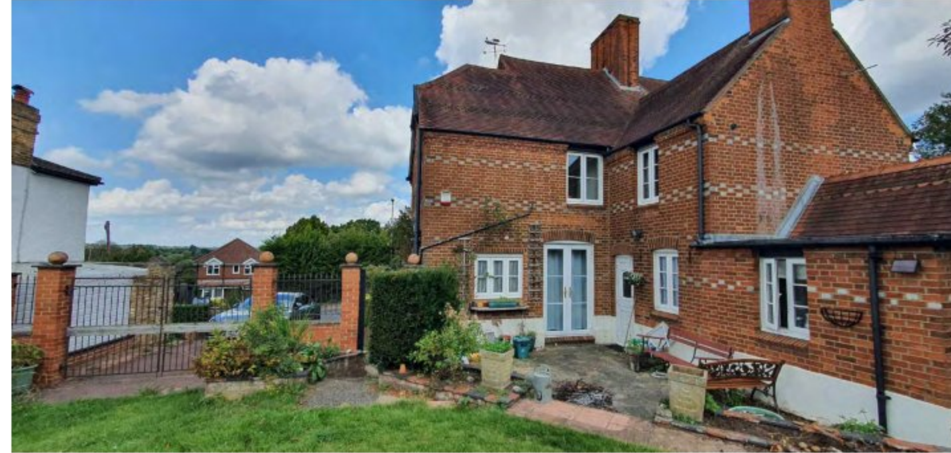
View of rear of existing house
