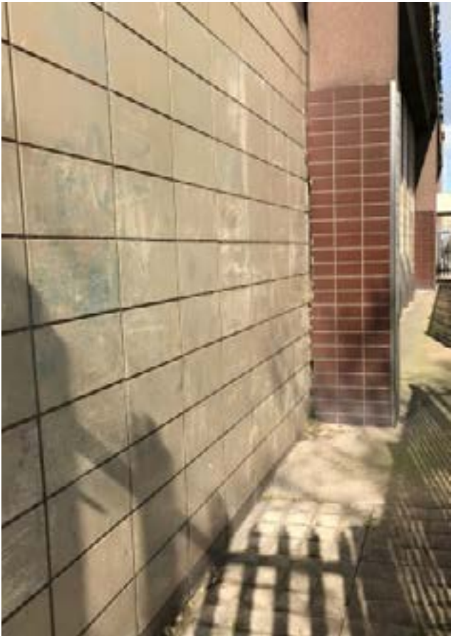
Figure 23. Glazed block colour and texture, with obvious graffiti damage
