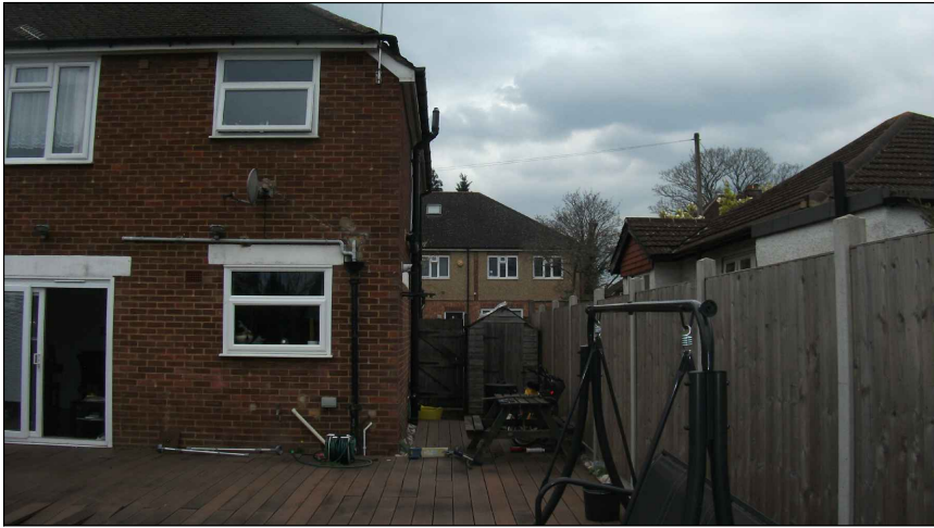
REAR PICTURE SHOWING BOUNDARY LINE WITH NUMBER 29
