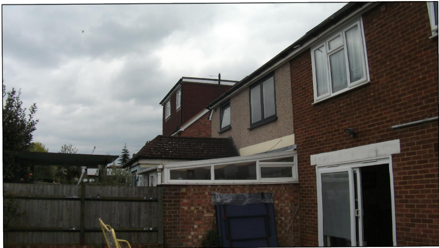
REAR PICTURE SHOWING BOUNDARY LINE WITH NUMBER 31
