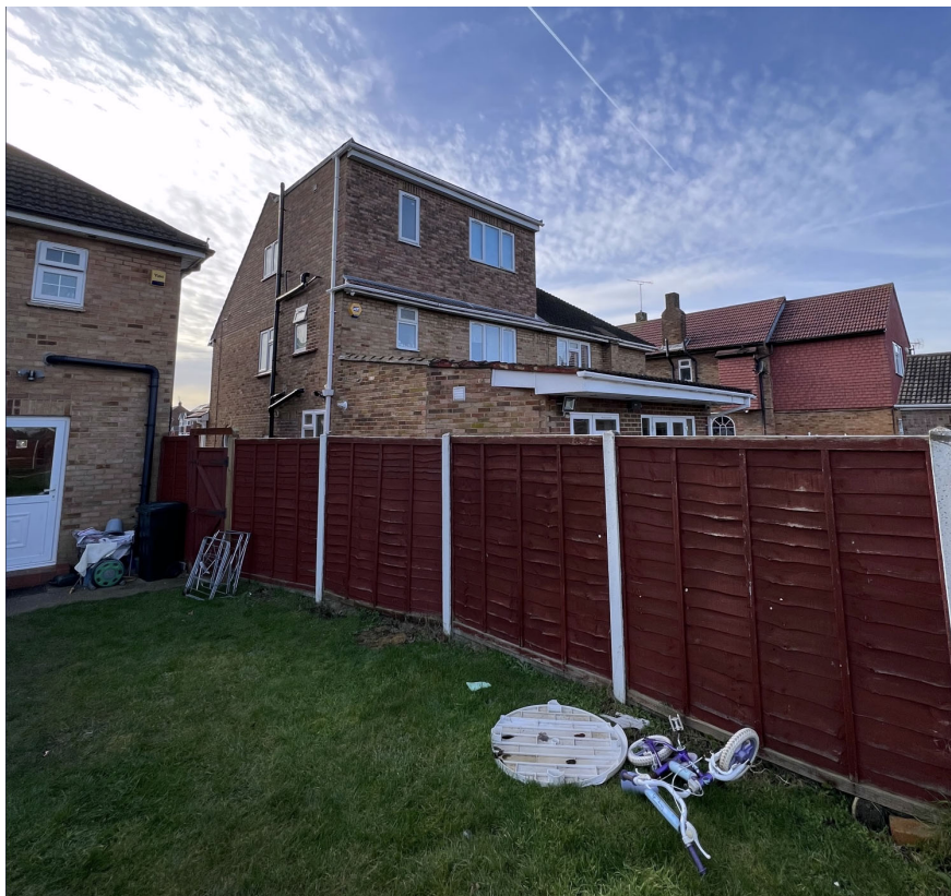
Rear of Neighbouring Property No. 15 Victoria Lane
