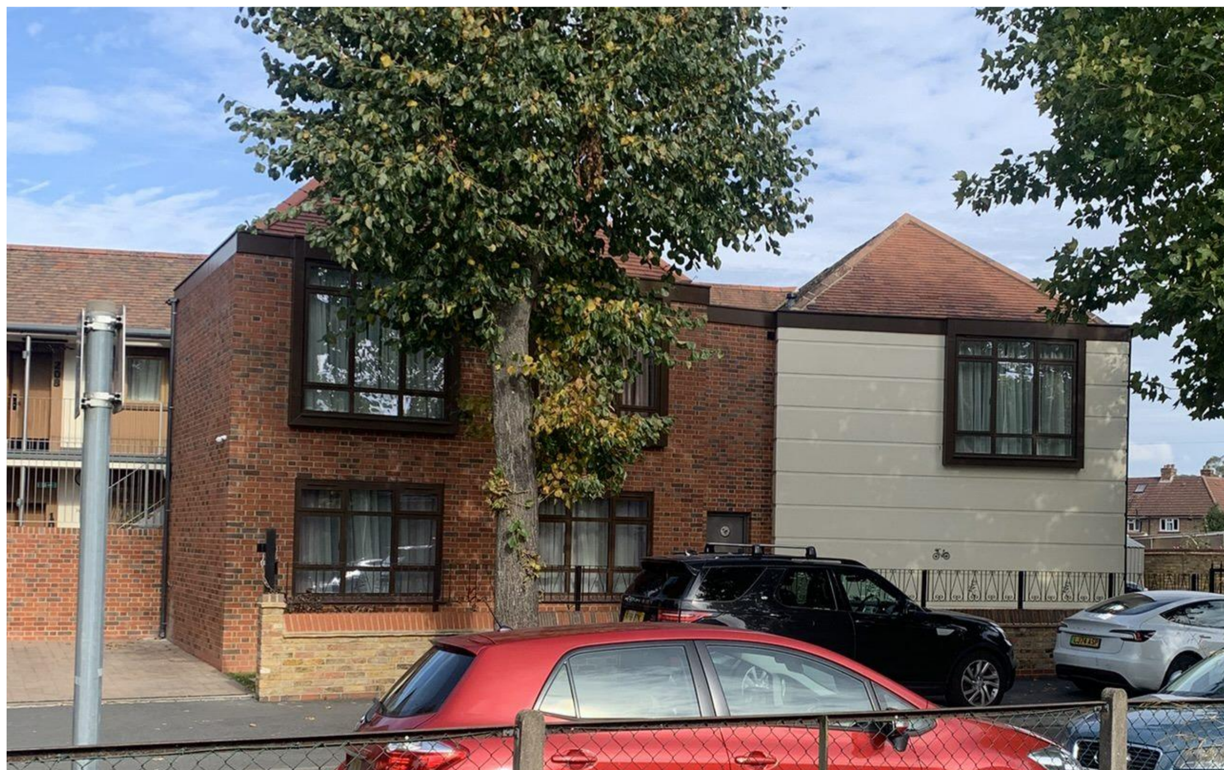
VIEW 2 AS EXISTING - PHOTO
