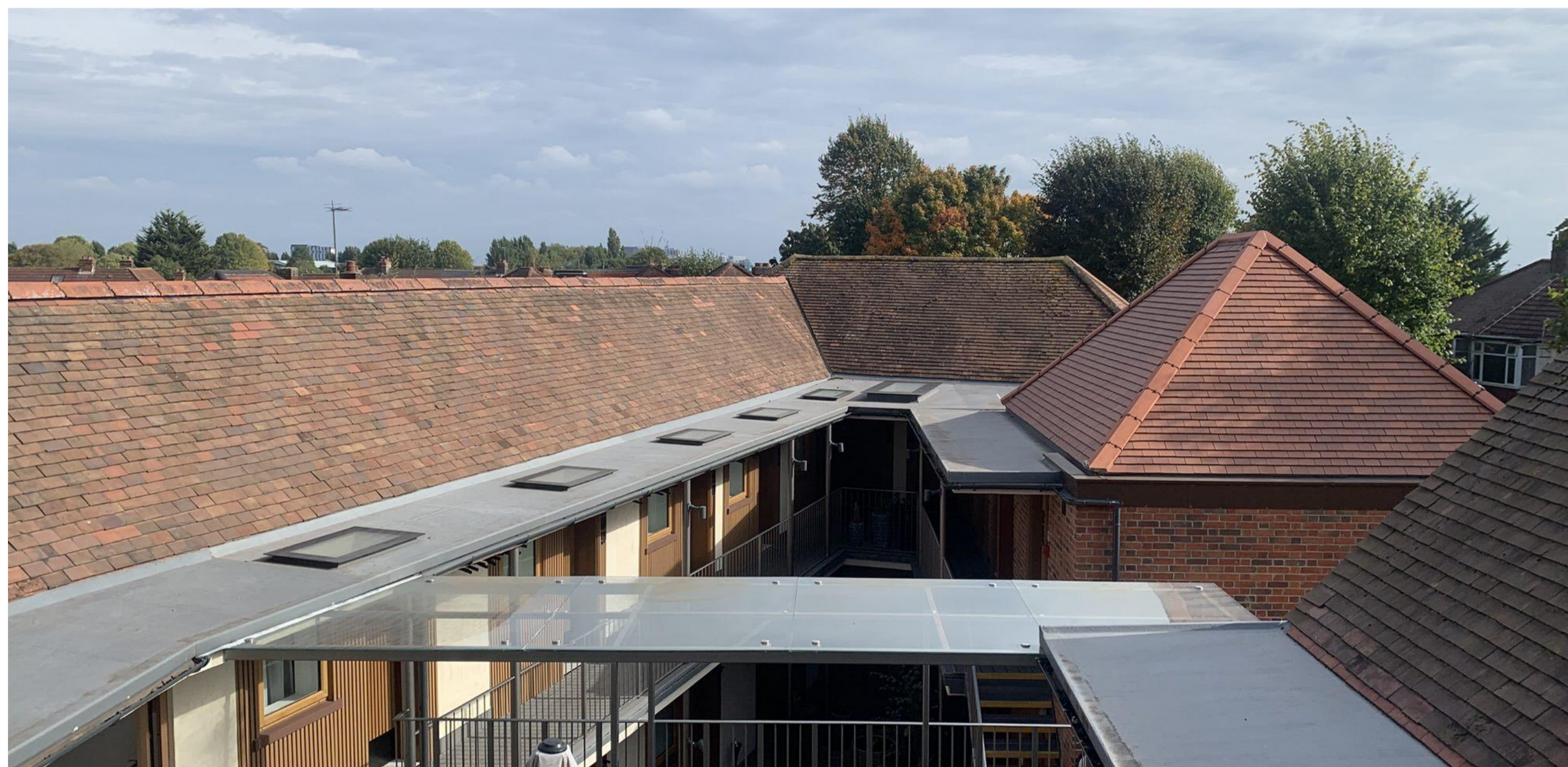
VIEW 1 AS EXISTING - PHOTO
