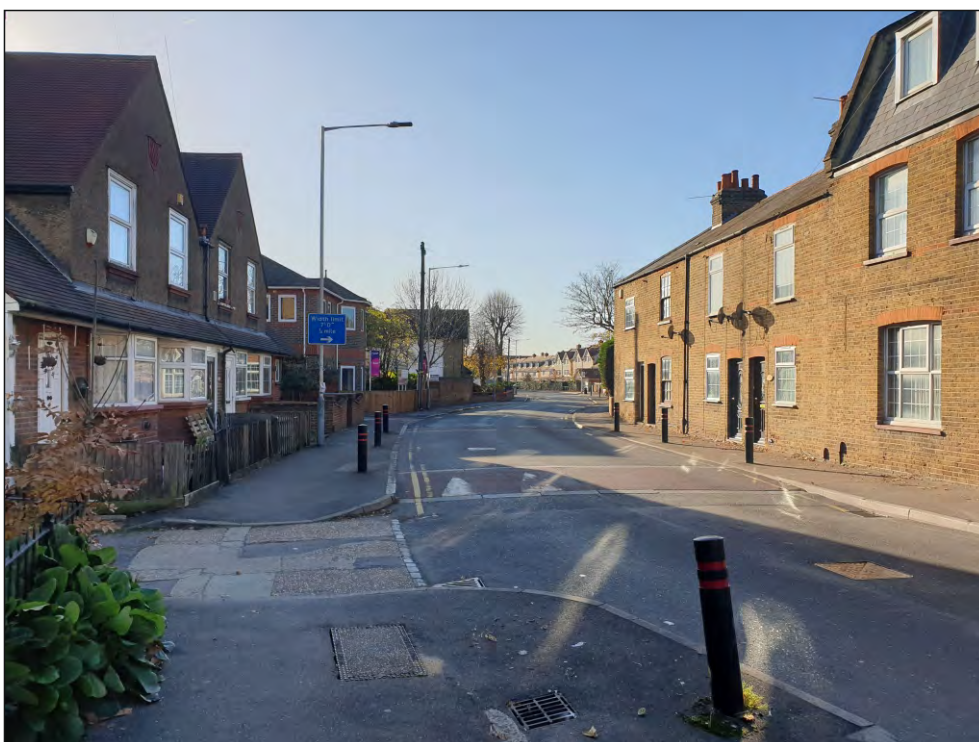
Pl. 18 General view of the Fountain House Hotel from the corner of Wistowe House showing views completely obscured by No. 220 Church Road. Looking south.
