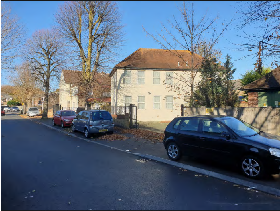
Pl. 7 General view of the Fountain House Hotel and the modern rear block from St Mary's Road. Looking northwest.
