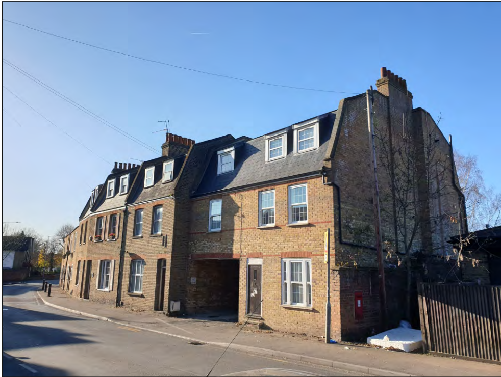
Pl. 19 General view of Nos. 221-233 Church Road (left) showing the relatively sympathetic modern development at Nos. 235-7 (centre) with regards to form, design and scale. Looking southwest.
