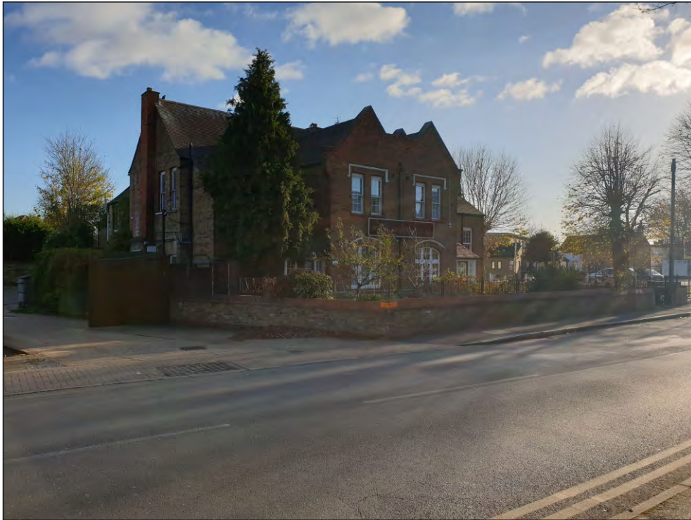
Pl. 3 General view of the Fountain House Hotel showing the yellow brick main block with its regular fenestration and projecting red brick chimney stack. Visible in the foreground is the former entrance porch with its modern lean-to extension. Looking southeast.
