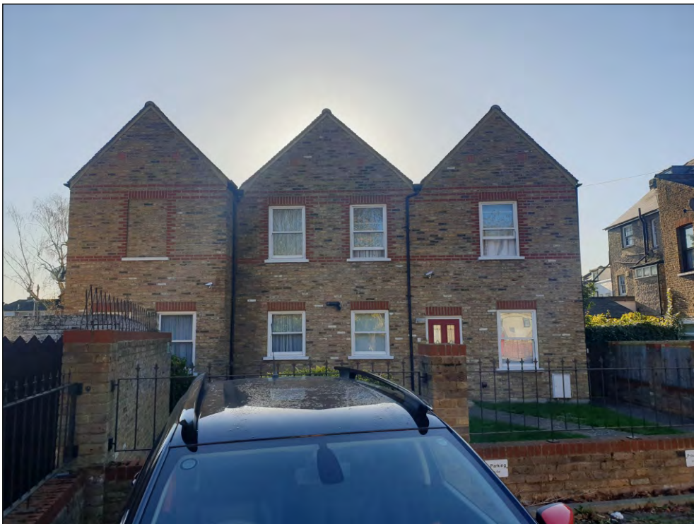
Pl. 20 General view of the modern development at Nos. 1-4 Butchers Mews. These buildings share a consistency with the neighbouring early 20th century properties with regards to form, design and scale. Looking south.
