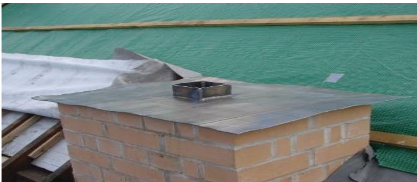
Image B: A chimney DPC is especially necessary where moisture penetration would be visually unacceptable and could damage the structure below
