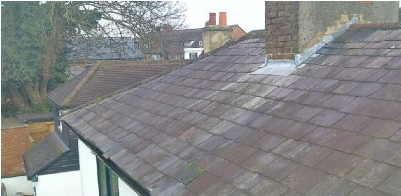
Left hand hip of slate roof covering
