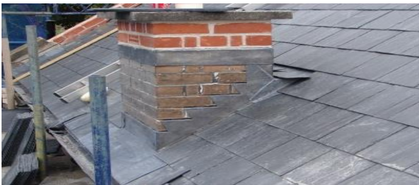
Image C: This image shows a chimney DPC, with correctly detailed step flashing, a back gutter and a front apron
