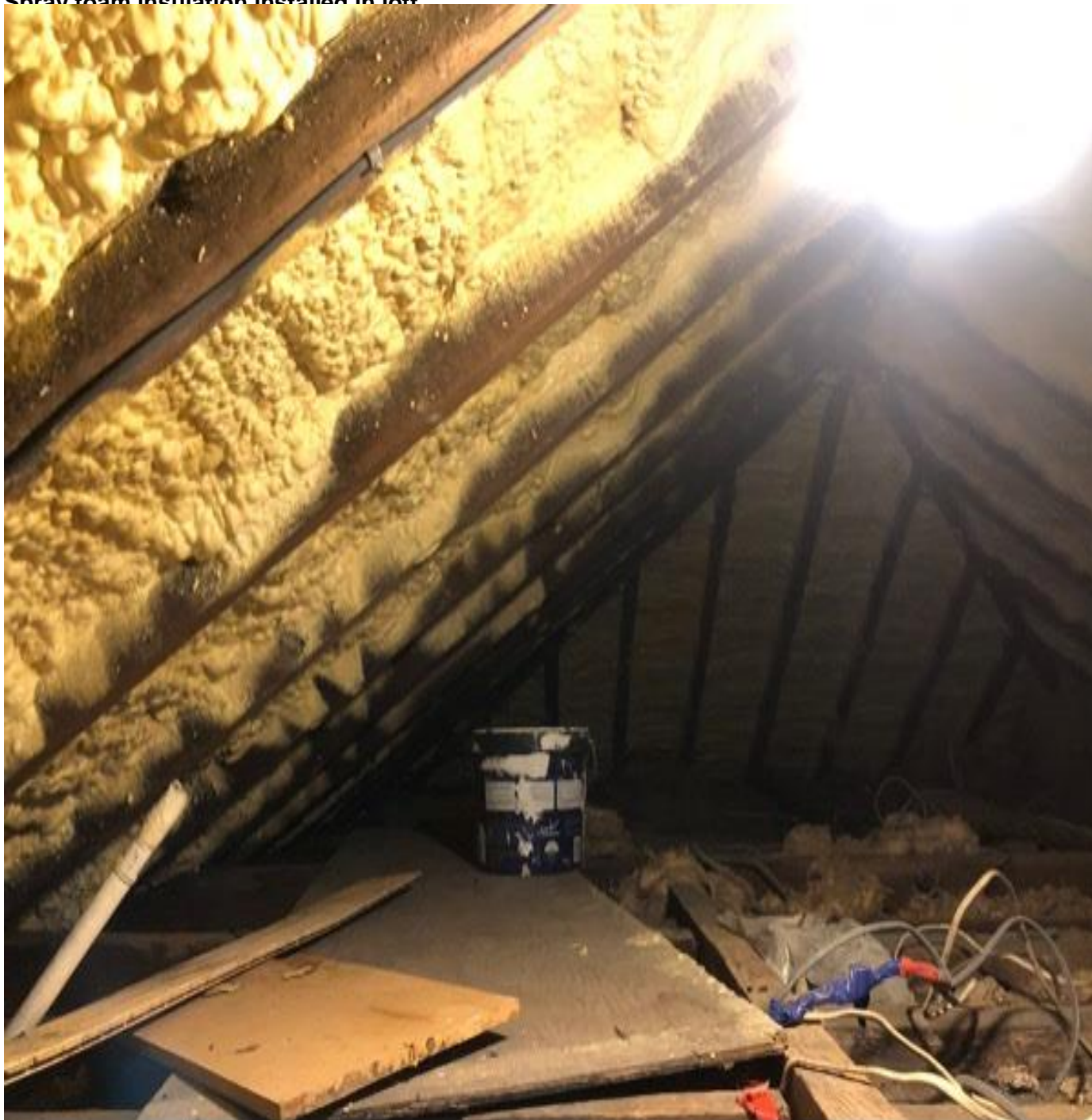
Spray foam insulation installed in loft
