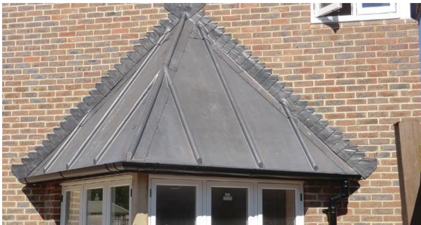
Bay window with stepped cavity tray
