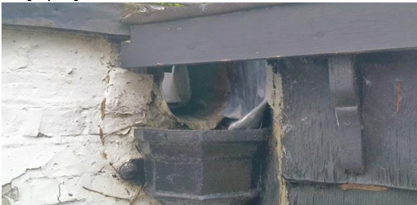
Front gulley and gutter rainwater outlet
