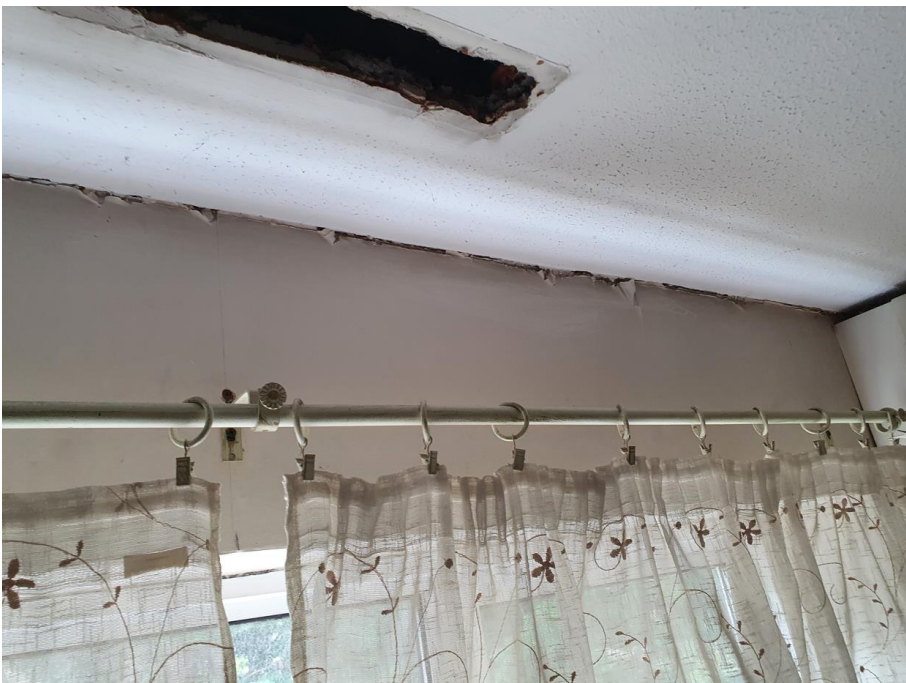
Gap at first floor rear bedroom between wall and ceiling
