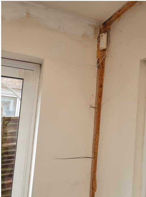
Infilled gap where conservatory is rotating away from original house
