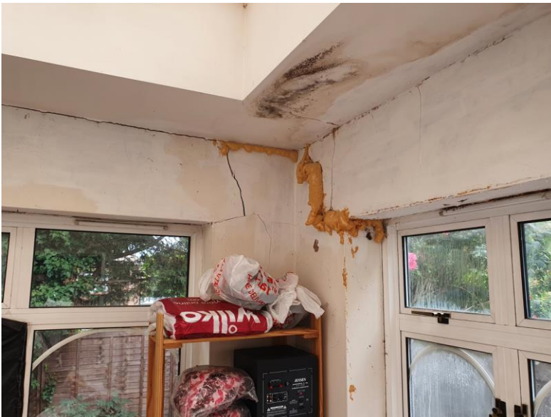
Cracking inside conservatory
