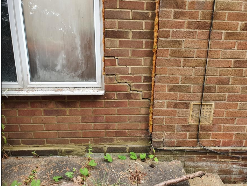
Cracking at rear of conservatory and infilled gap at joint with main house
