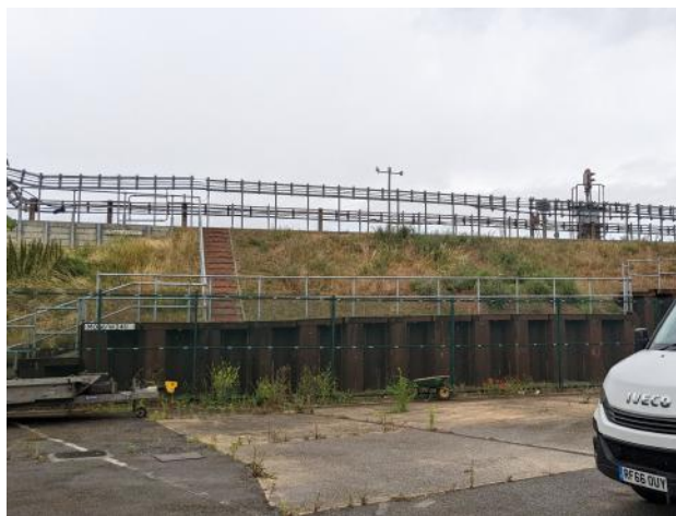
Photograph Three: Retaining wall (sheet piles) and railway line to rear / south of site
