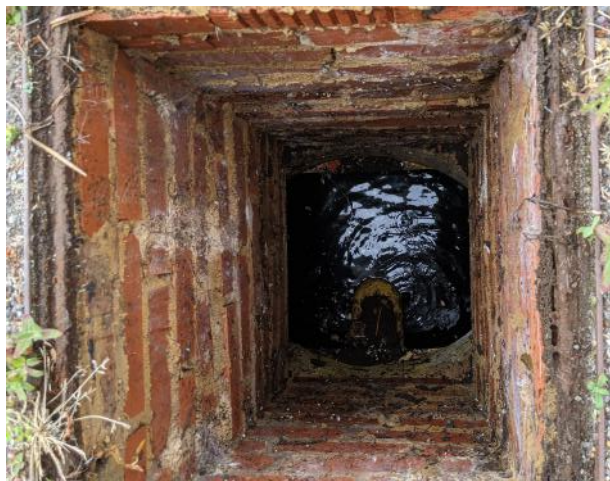
Photograph Four: Middle chamber of drainage interceptor.
