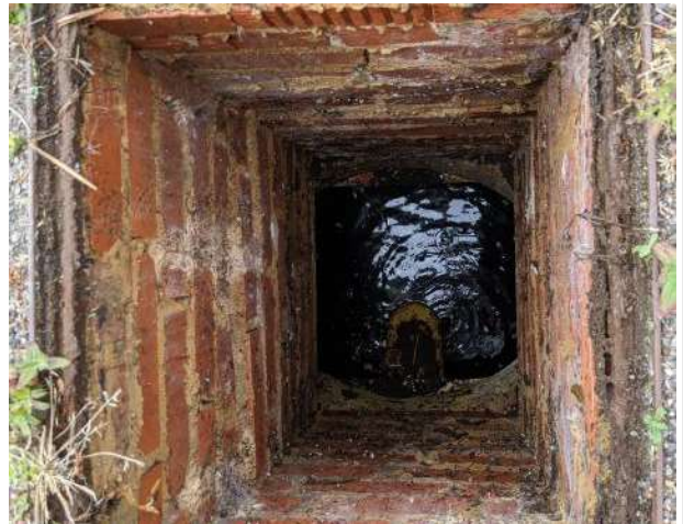
Photograph Four: Middle chamber of drainage interceptor.
